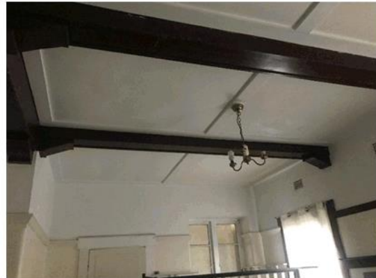
Figure 40 – Interior fabric, third floor apartment ceiling detailing with batten over plaster sheeting and expressed timber beams with original shellac finish.
