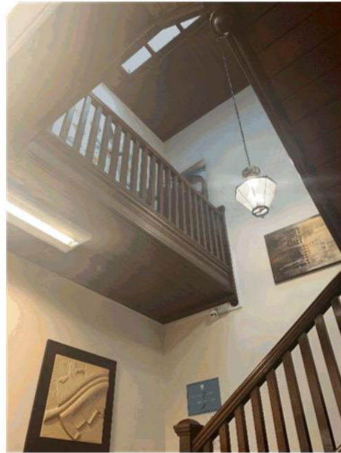
Figure 106 – Detail of timber tongue-and-groove soffit to stair and skylight above.
