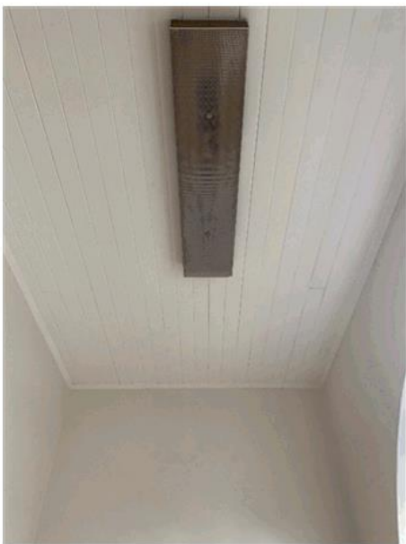
Figure 116 – Timber tongue-and-groove ceiling in enclosed veranda space.
