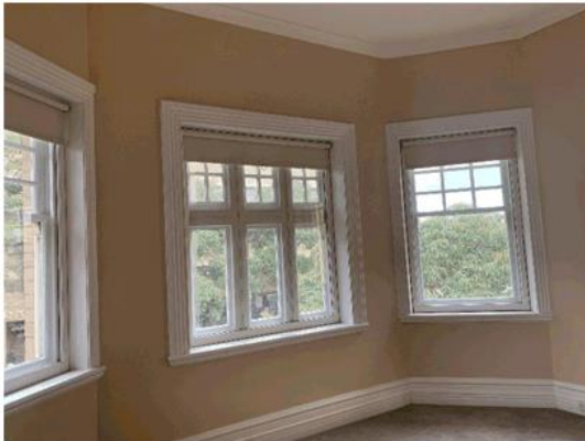
Figure 76 – First floor, timber-framed bay window in south-western room (all windows have later addition secondary frame for acoustic screening).
