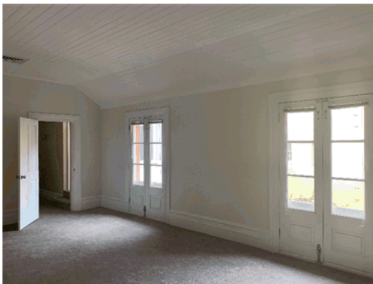
Figure 86 – First floor, northern room – note timber tongue-and-groove ceiling.
