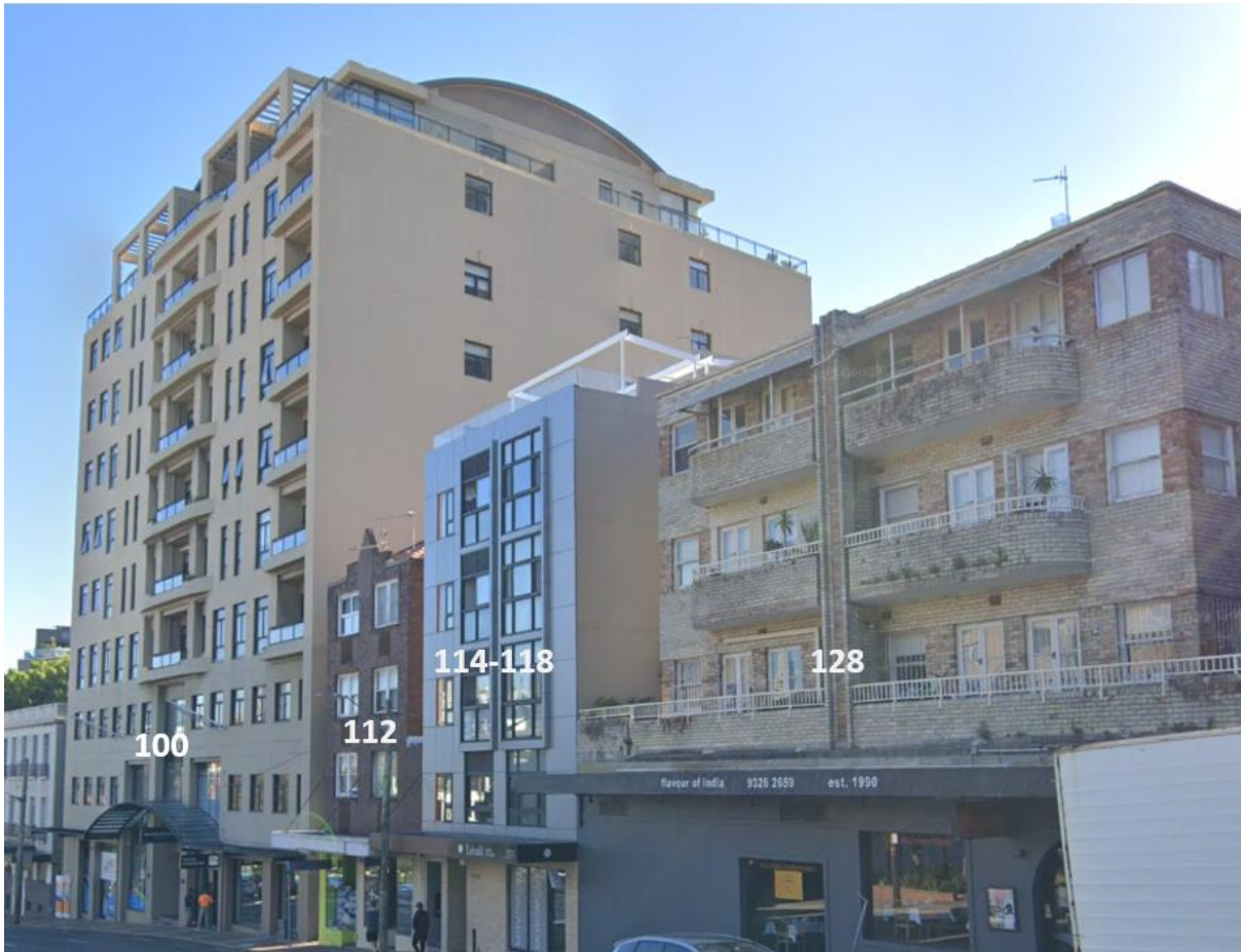
Figure 8: Nearby apartment buildings at 100-128 New South Head Road (to the south of the subject site) on the northern side of New South Head Road
