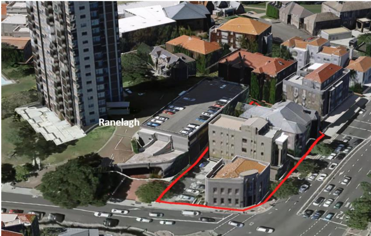
Figure 4: 3D view of site at 136-148 New South Head Road, Edgecliff (Source: Council Maps)
