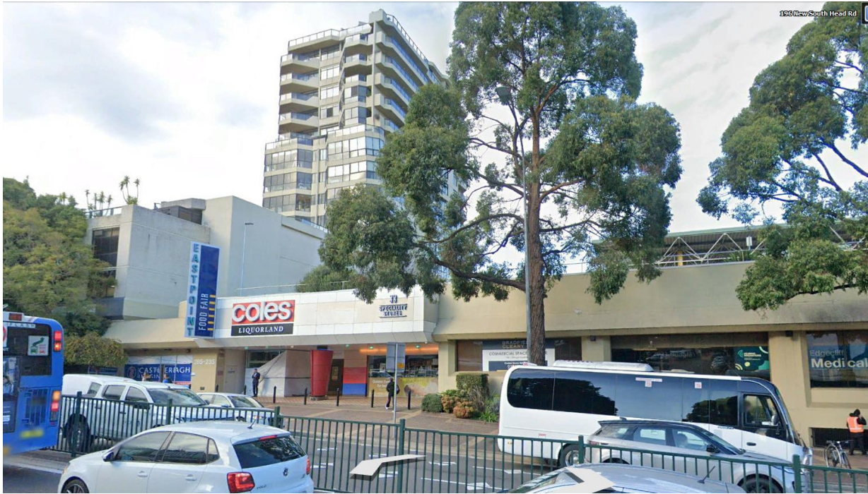
Figure 10: View of the Eastpoint Food Fair at 238-285 New South Head Road, the bus and rail interchange and the Eastpoint Tower behind
