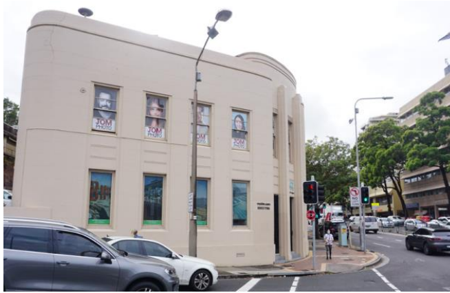
Figure 4 – Existing heritage listed commercial building
