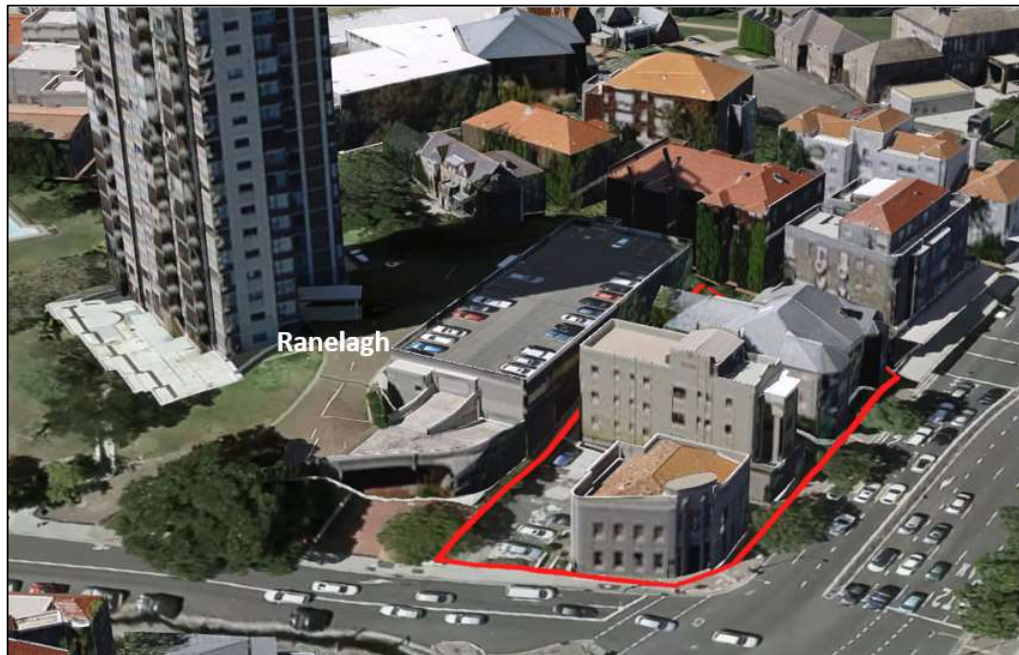
Figure 5: 3D view of 136-148 New South Head Road (with the site highlighted in red) viewed from the west.
