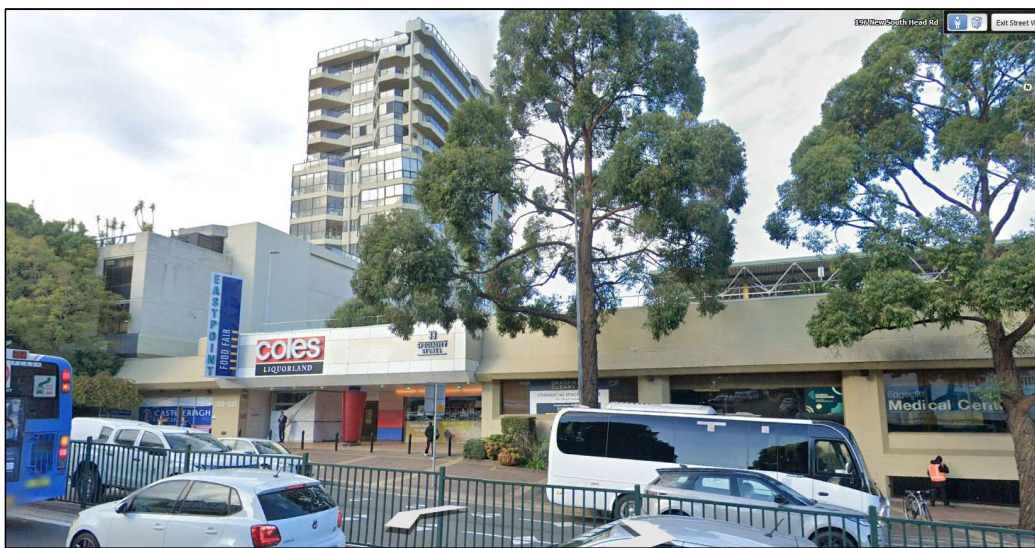
Figure 11: View of the Eastpoint Food Fair at 238-285 New South Head Road, the bus and rail interchange and the Eastpoint Tower behind
