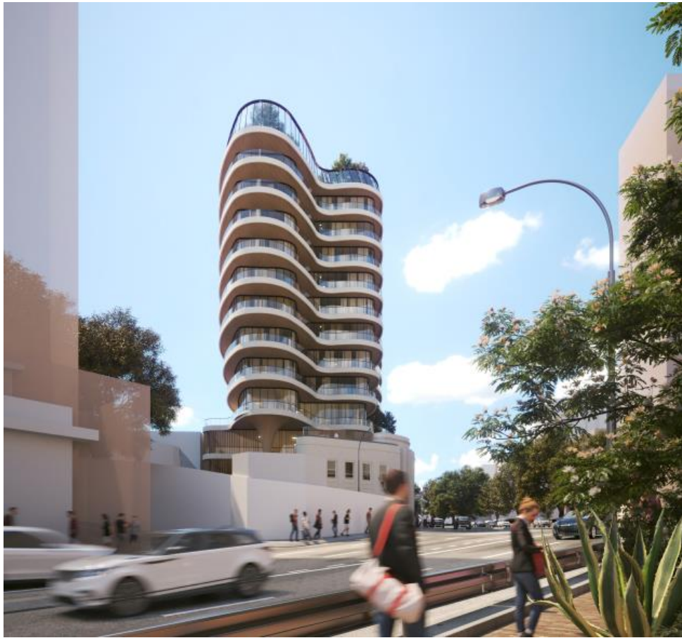
Figure 1 – Photomontage of concept building viewed from New South Head Road to the east
