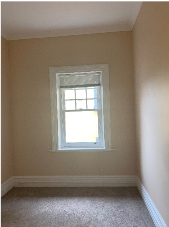
Figure 78 – First floor, showing original timber framed double-hung sash window and skirting.
