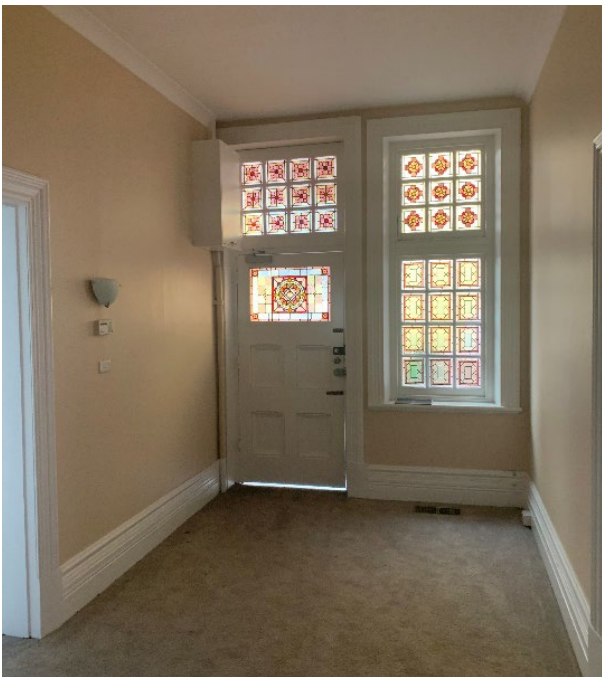
Figure 60 – Main door entry, internal view. Original timber architraves and stained-glass panel fanlights and side lights.
