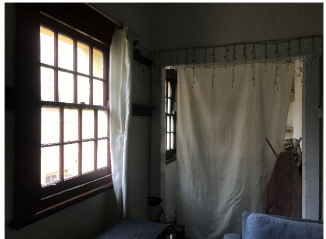
Figure 38 – Interior fabric third floor apartment windows and alcove.
