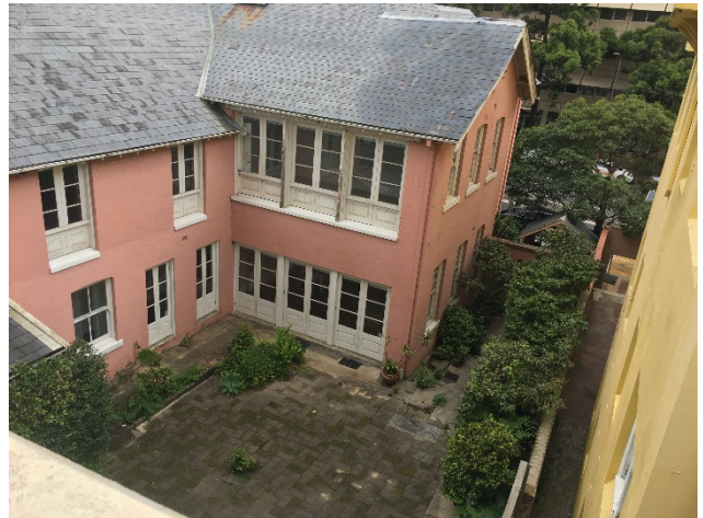
Figure 58 – Rear (north-western side) of property, showing rear elevations with altered window openings extended to create full length windows and French doors.
