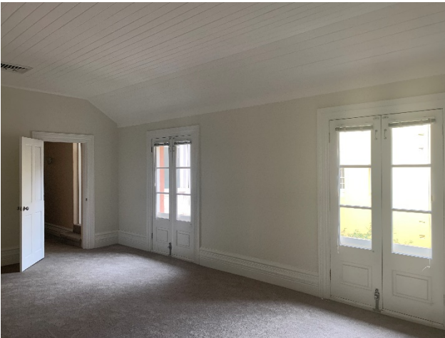
Figure 86 – First floor, northern room – note timber tongue-and-groove ceiling.
