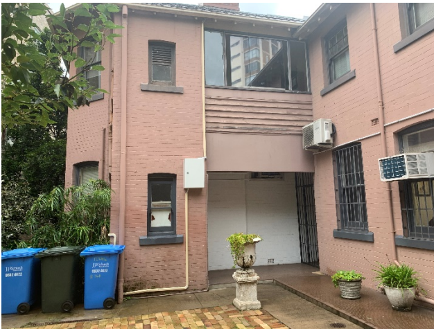
Figure 96 – North-eastern façade, ground-floor level. Note secondary bay at left of image.
