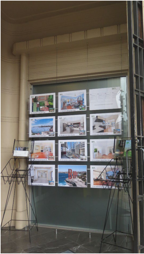
Figure 11 – Main entry door enclosed with glazed infill
