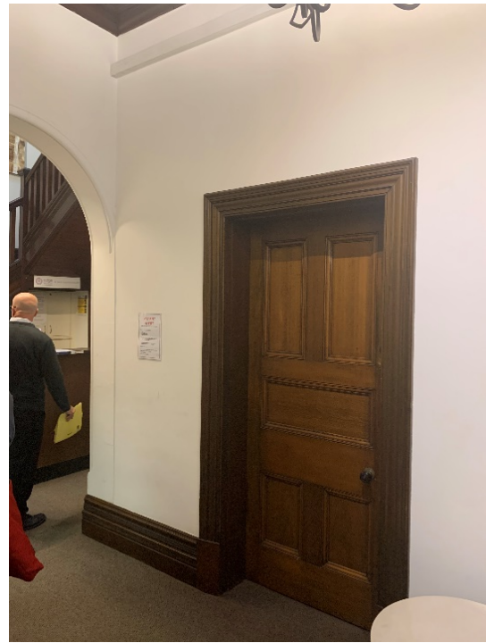
Figure 102 – Timber panel door to room off main hallway (common foyer).
