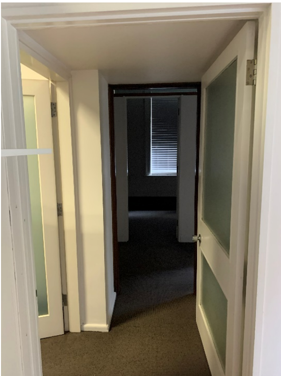
Figure 119 – Ground-floor, showing subdivided rooms in southern portion. False ceilings installed.
