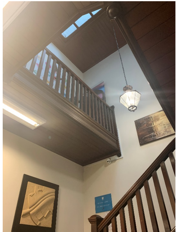
Figure 106 – Detail of timber tongue-and-groove soffit to stair and skylight above.
