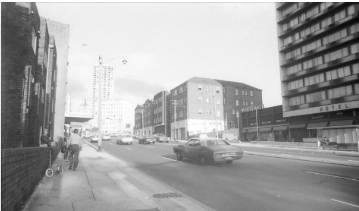
Figure 157 - New south Head Road, facing east. Apartment complex tower Ranelagh visible in background
