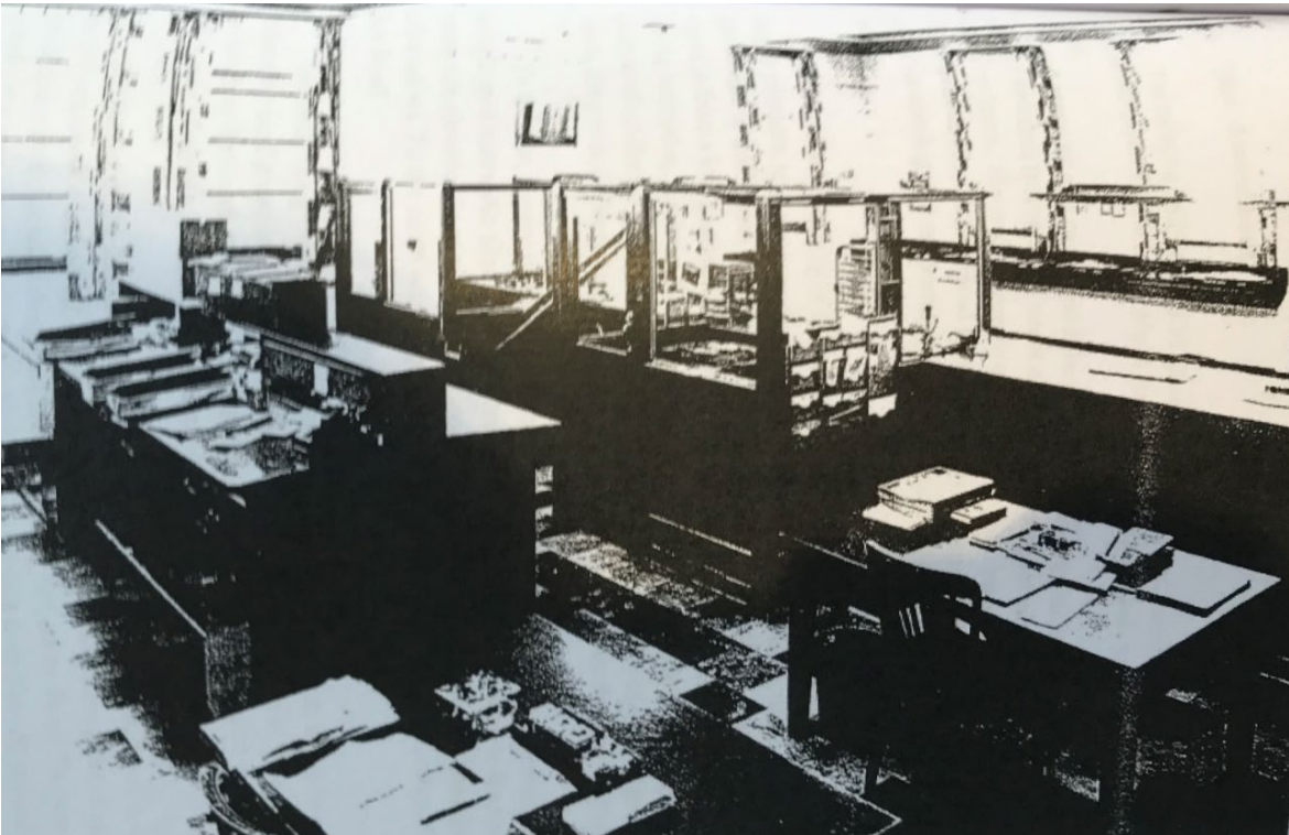
Figure 137 – Interior of ground floor banking chamber, June 1959.
