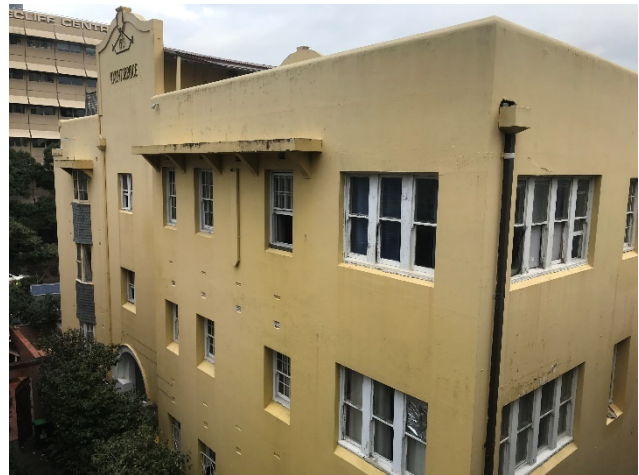
Figure 30 – View of eastern façade with concrete awning over upper windows. The corner windows appear to be later addition infilled balconies.
