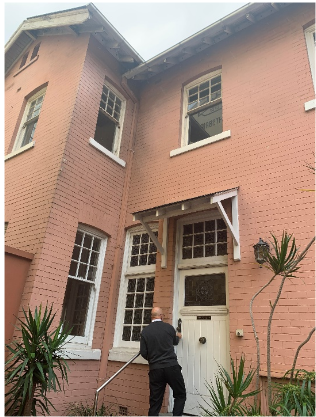
Figure 54 – Main entrance to building on west elevation.
