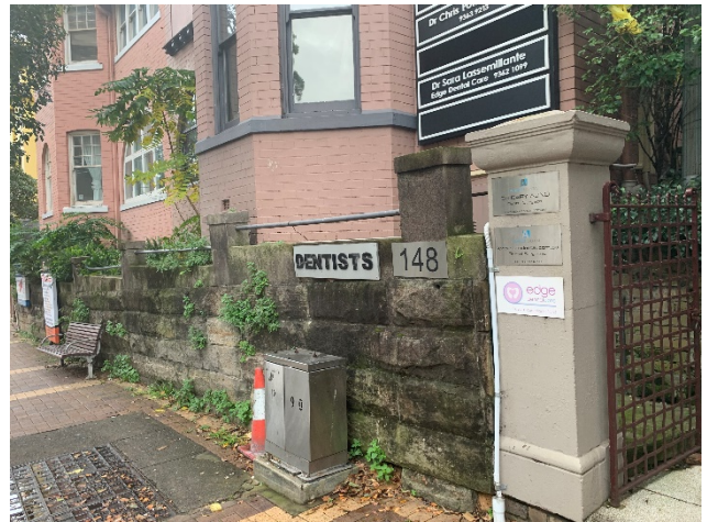
Figure 89 – Detail of rusticated sandstone boundary wall, which runs across 142-148 New South Head Road where the semi-detached properties sit.
