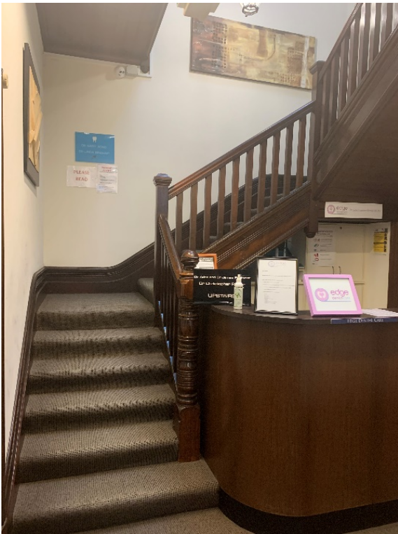
Figure 105 – Timber stair at western side of ground-floor.
