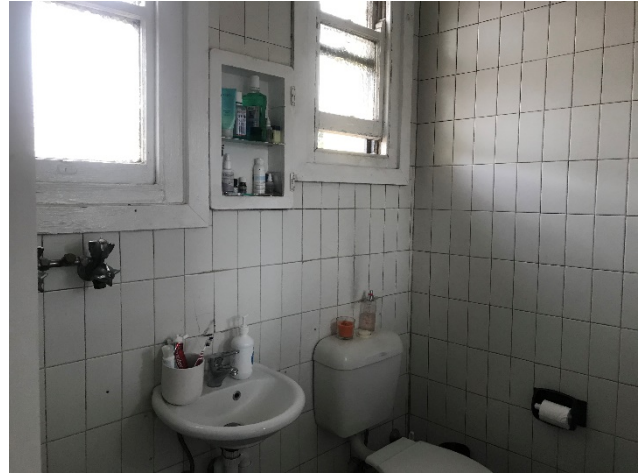
Figure 46 – Bathroom fabric with later addition fitout
