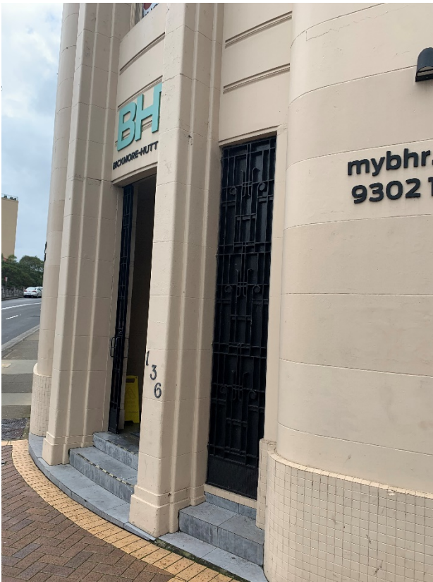
Figure 9 – Main entrance to ground floor banking chamber with metal grilles.
