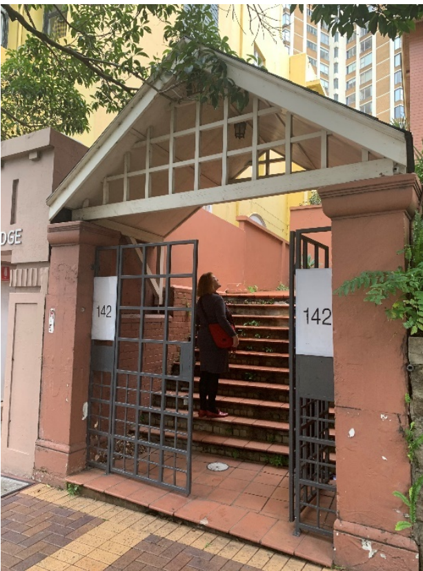
Figure 53 – Entrance gate and stairs from New South Head Road.
