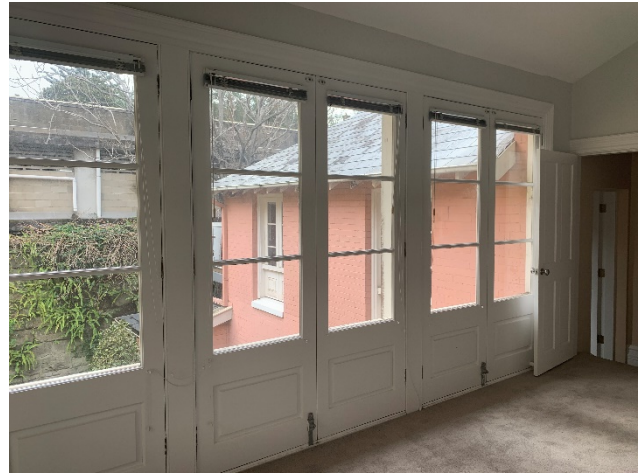
Figure 85 – First floor, north-western room, later addition French doors and enclosed former verandah.
