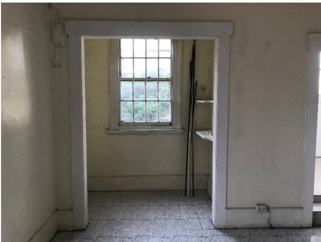
Figure 37 – Interior fabric, third floor apartment alcove with multipaned, double-hung sash windows.
