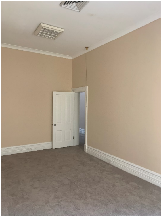
Figure 80 – First floor, large-format north-western room with later addition plasterboard ceiling.
