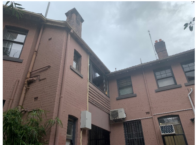
Figure 95 – Detail of fenestration at upper level of building rear.
