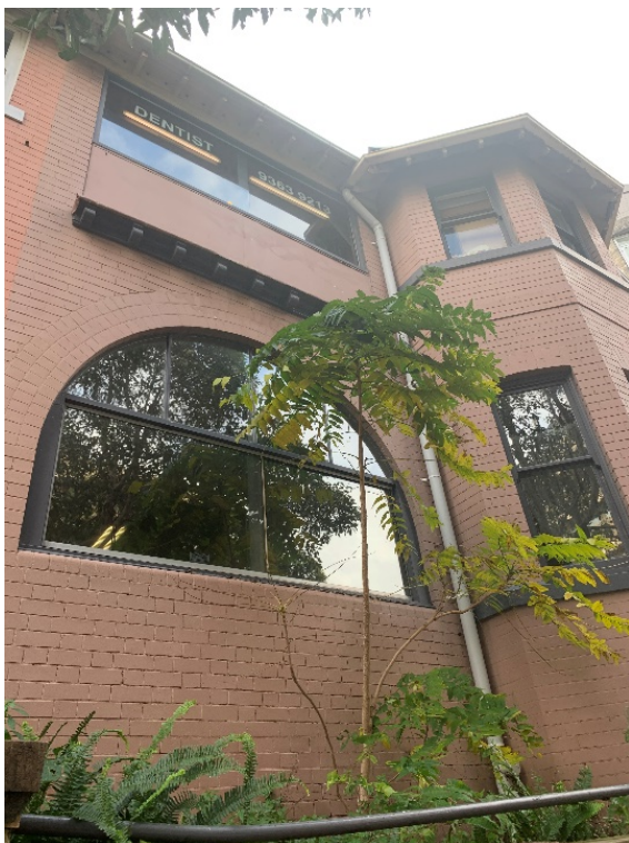
Figure 90 – Detail of south elevation to New South Head Road. Note the enclosed verandah to ground and first floors.
