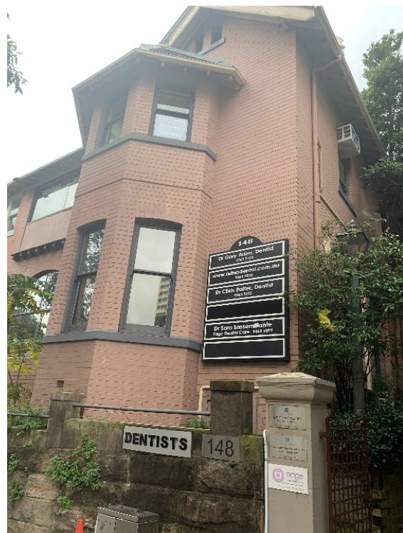
Figure 91 – Detail of faceted bay at south-eastern corner, abutting face brickwork gabled wall to New South Head Road. Brickwork has been painted.
