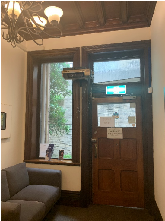
Figure 101 – Main entry foyer, internal view showing timber door and window architraves, skirting and ceiling with shellac finish. Later addition front door and timber panel ceiling. Stained glass removed and windows modified.
