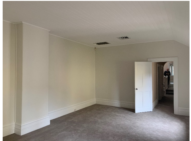
Figure 87 – First floor, northern room – note chimney breast along eastern wall.
