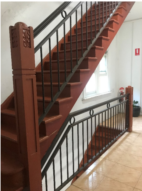
Figure 49 – Stairwell and staircase with simple decoration to newel post and metal balustrading.
