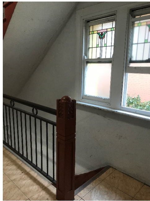
Figure 50 – Stairwell, window and timber staircase and stained-glass window to upper sash.
