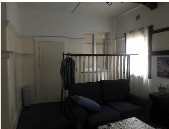
Figure 41 – Interior fabric, view of enclosed balcony, third floor apartment.
