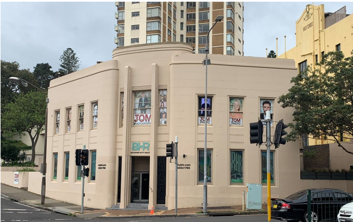
Figure 13 – View of No 136 showing the curved form of the painted rendered masonry walls with horizontal banding to spandrel panels, parapets and other decorative elements
