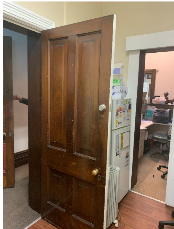
Figure 108 – Timber door to treatment room under stair.
