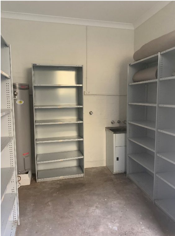
Figure 68 – Ground-floor, single-storey laundry and store wing extension with concrete slab floor.
