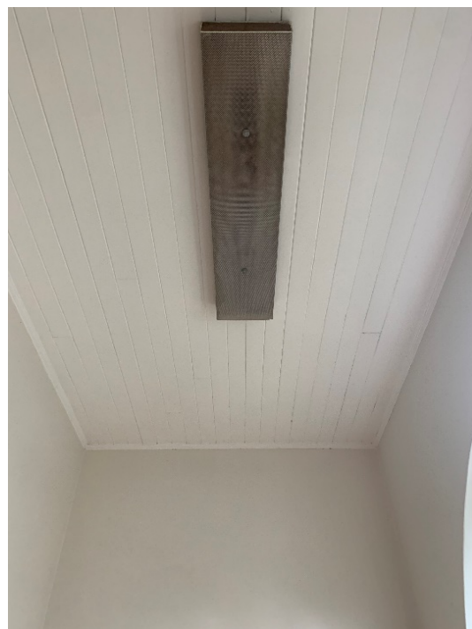
Figure 116 – Timber tongue-and-groove ceiling in enclosed veranda space.
