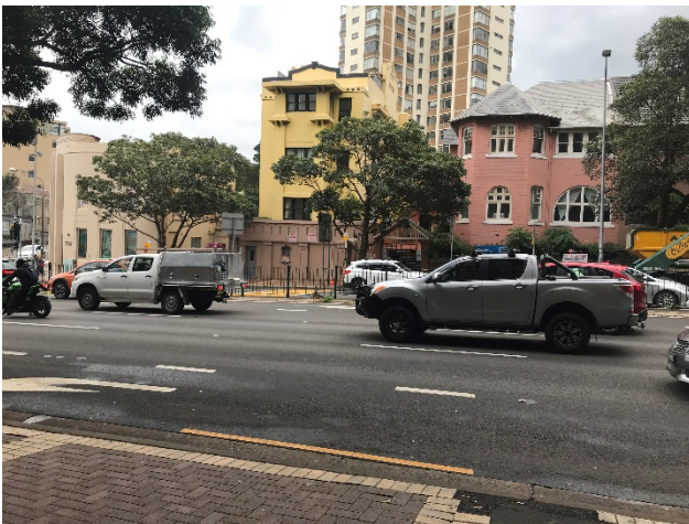
Figure 27 – View of southern façade fronting New South Head Road.
