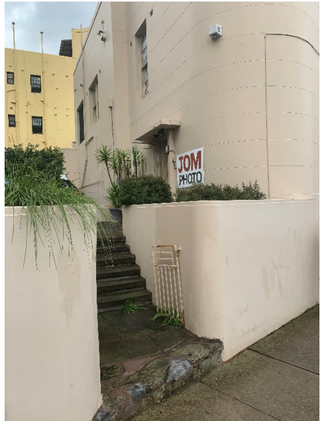
Figure 12 – Side entrance from Darling Point Road.
