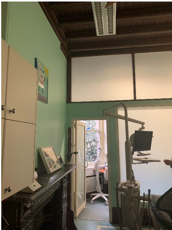
Figure 111 – Treatment room at eastern side of ground-floor, facing east towards partition wall.
