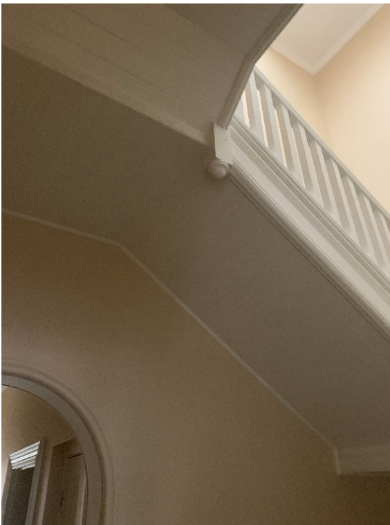
Figure 70 – Detail of painted, timber tongue-and-groove soffit to stair.
