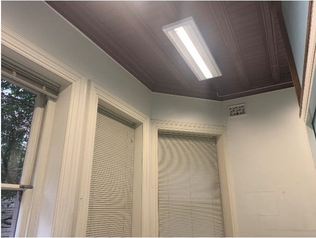
Figure 113 – Bay window located on east elevation of ground-floor treatment room.
