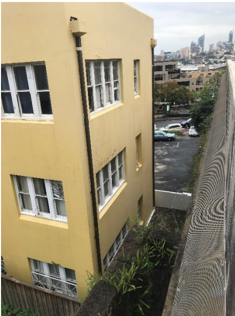
Figure 31 – View of northern façade and sandstone flagging at rear of building.
