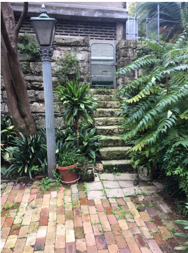
Figure 98 – Sandstone steps and boundary wall at north-eastern corner of the property.
