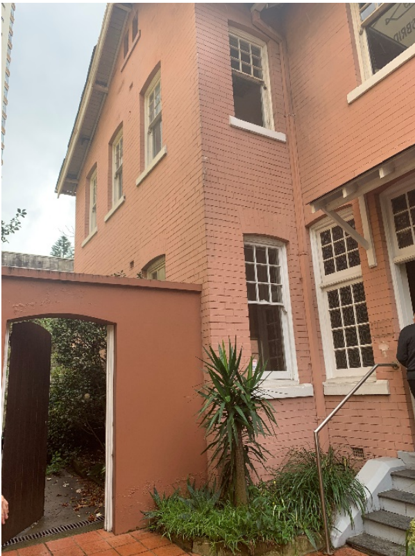
Figure 55 – Western elevation with later addition painted brickwork.
