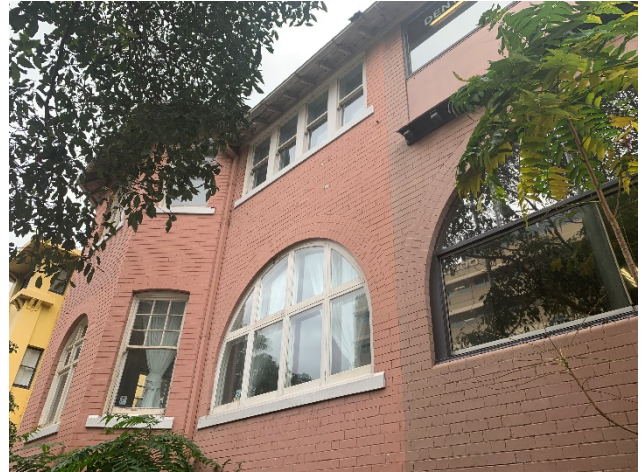
Figure 52 – Detail of principal elevation to New South Head Road showing later addition infilled verandahs.
