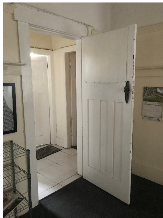
Figure 44 – Interior fabric, third floor apartment, with timber panel door.
