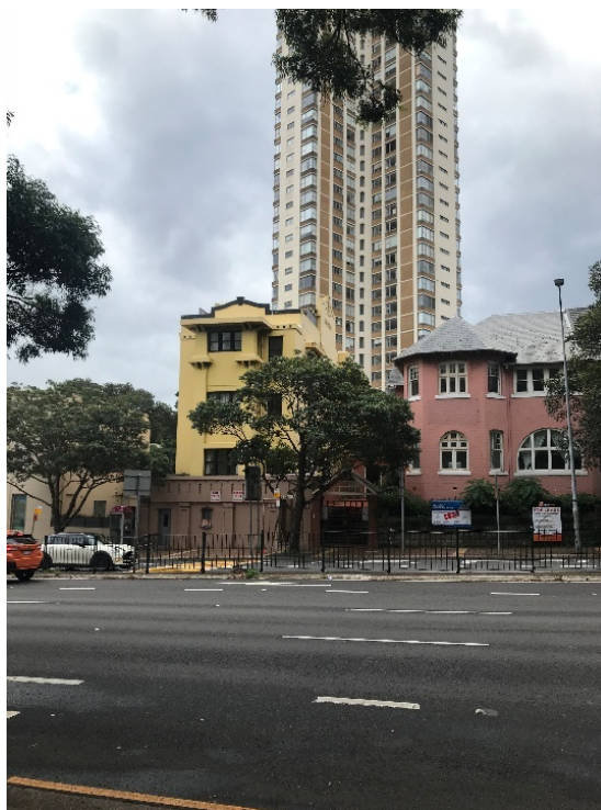
Figure 4 – View of subject sites from southern side of New South Head Road with apartment tower visible behind.
