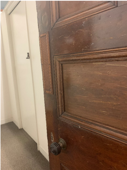
Figure 103 – Detail of original timber door with finger pad.
