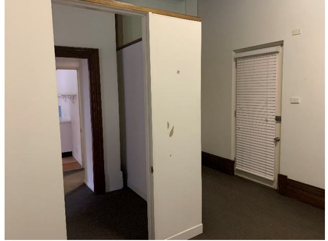
Figure 122 – Lightweight partition screens at southern portion of ground floor.
