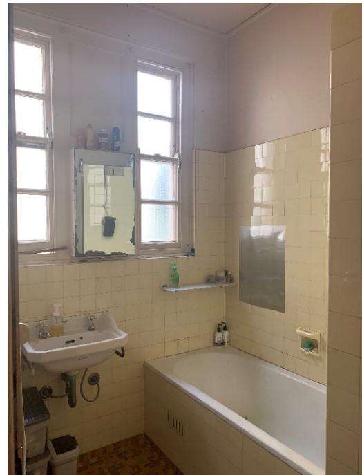
Figure 22 – Internal bathroom to first floor apartment.
