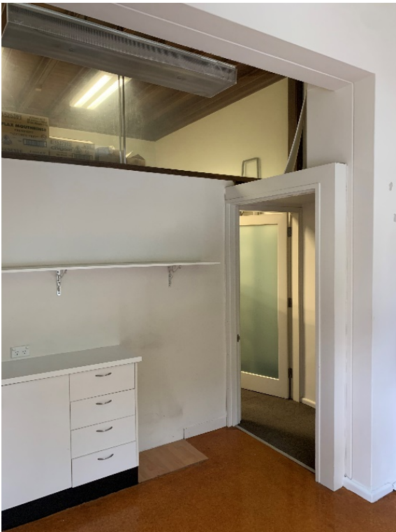
Figure 117 – Sub-divided spaces in southern portion of the building. Lightweight partitions.
