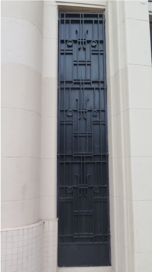
Figure 14 - Original decorative metal grille over window
