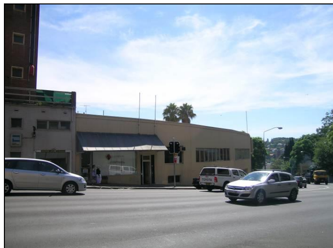
Photograph 1: The Subject Site, as viewed from New South Head Road.
