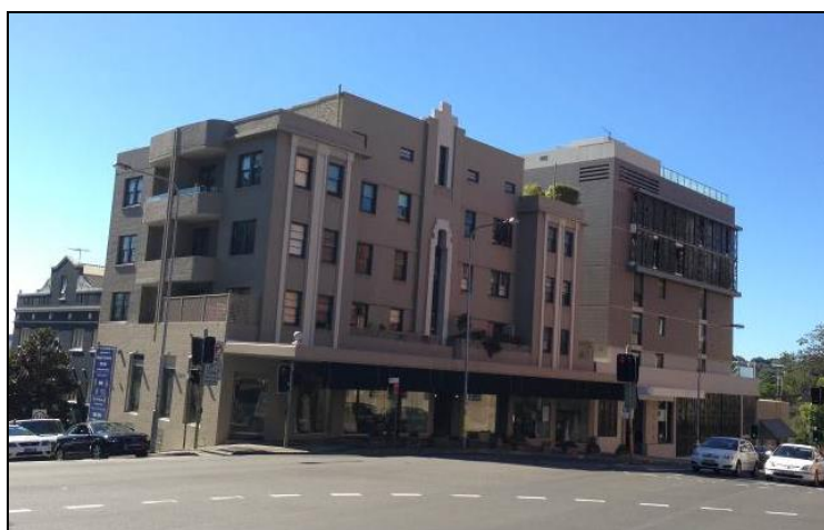
Photograph 9: Development to the west Nos. 220-238 New South Head Road.
