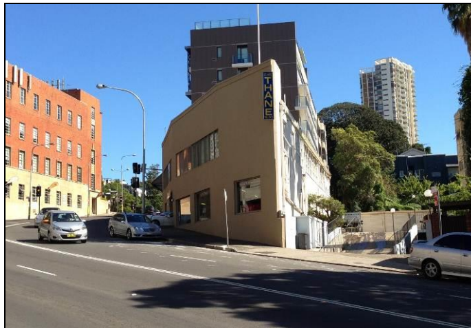
Photograph 2: The Subject Site, as viewed from New South Head Road.
