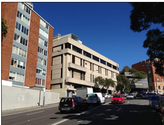
Photograph 8: Development to the south Nos. 297-299 New South Head Road.
