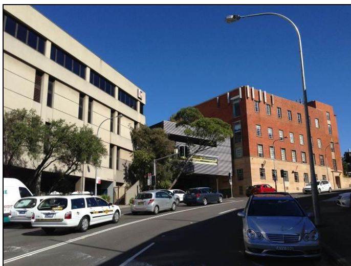
Photograph 7: Development to the south Nos. 289 New South Head Road.
