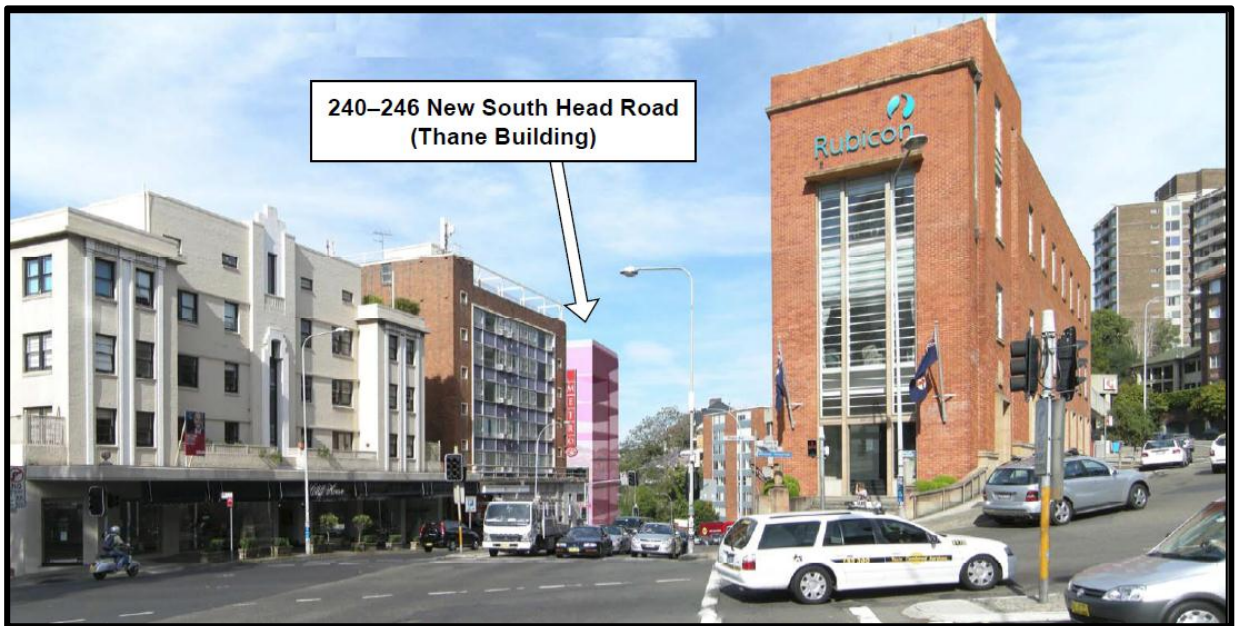
Figure 3: Photomontage of the 3D model - looking east from the corner of Ocean Street and New South Head Road
