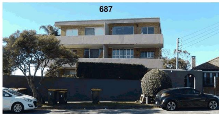
Figure 14: Existing development at 687 Old South Head Road, opposite the site in Waverley LGA, showing a 3 storey residential flat building
