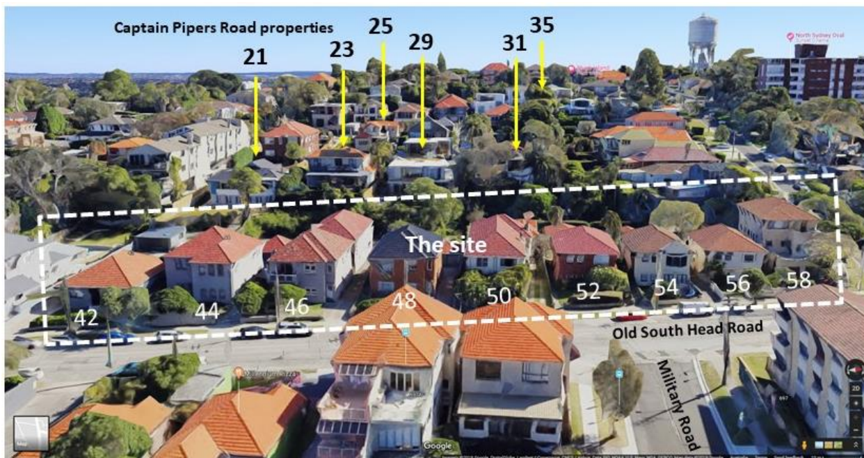
Figure 2: 3D digital model image of the site in relation to 21, 23, 25, 29, 31 and 35 Captain Pipers Road, Vacluse
