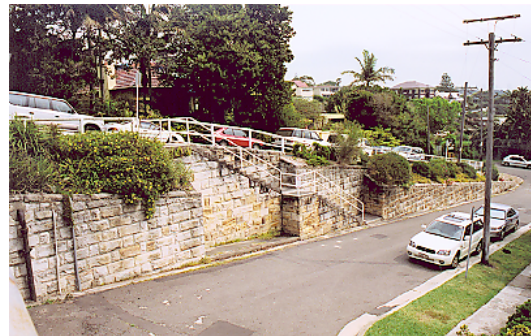
FIGURE 91 Significant sandstone retaining wall
