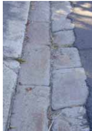
Sandstone guttering
