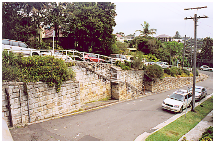
Sandstone retaining wall along Salisbury Street
