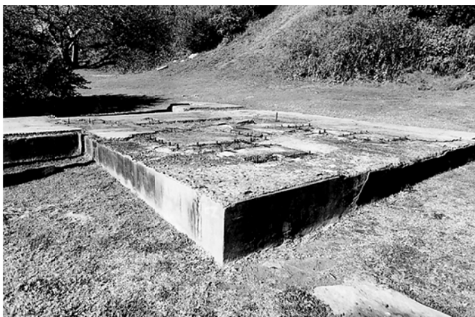
FIGURE 154 Concrete base to the boom-winch house
