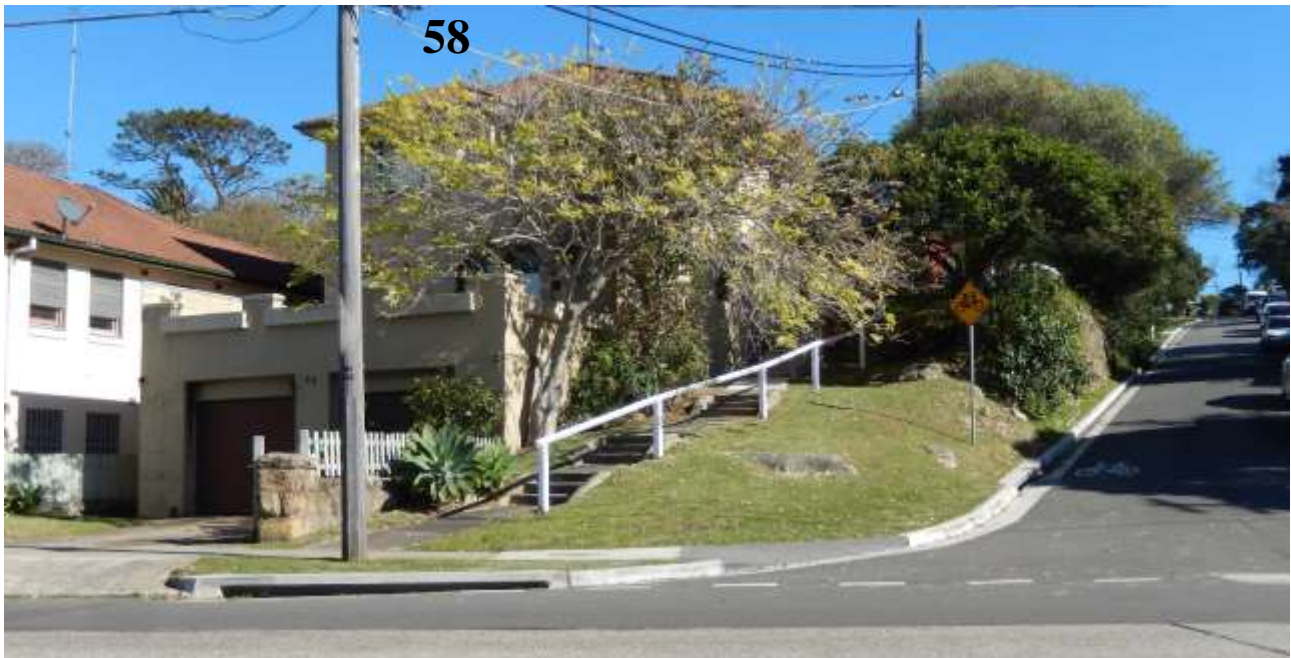
Figure 10: Existing development at 58 Old South Head Road showing Clarendon Street, public stairs and steep topography of site and surrounds
