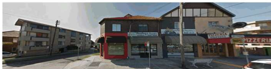
Figure 8: View of development opposite the site to the east (Source: Google Street View)
