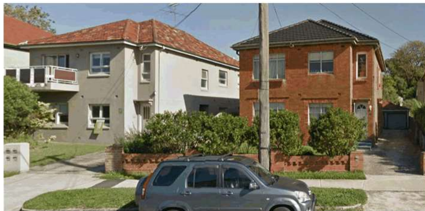
Figure 6: View of the subject site 46-48 Old South Head Road (Source: Google Street View)
