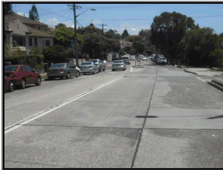
Photo 3: Old South Head Road at the subject site - facing north
