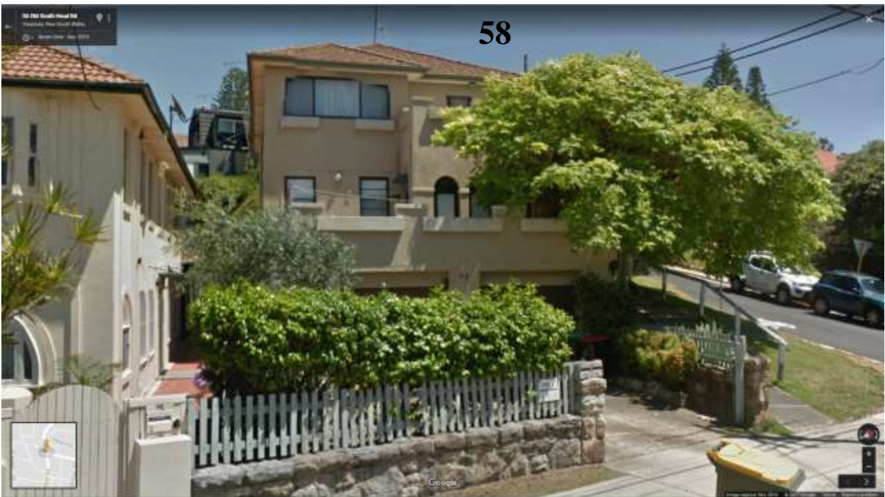
Figure 9: Existing development at 58 Old South Head Road (source: Google Maps)
