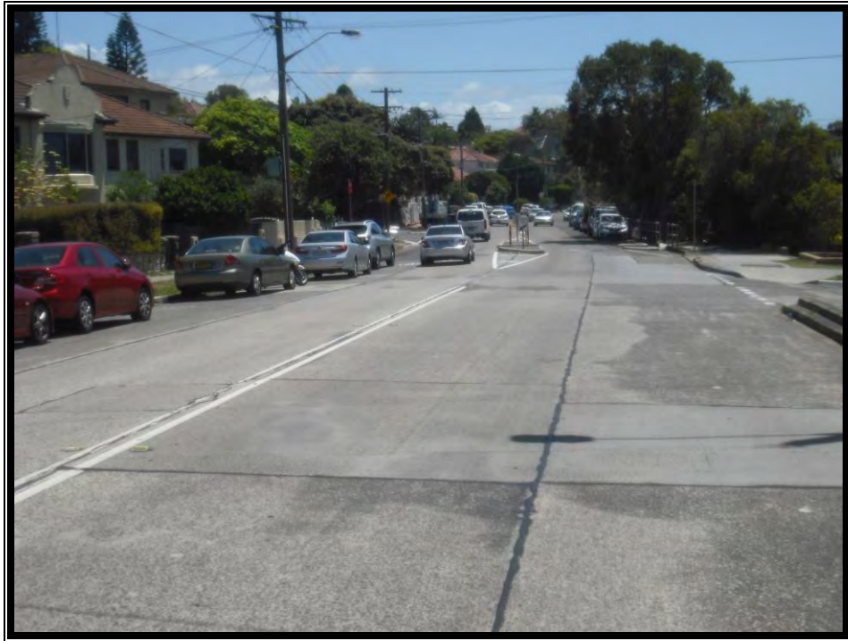
Photo 3: Old South Head Road at the subject site - facing north
