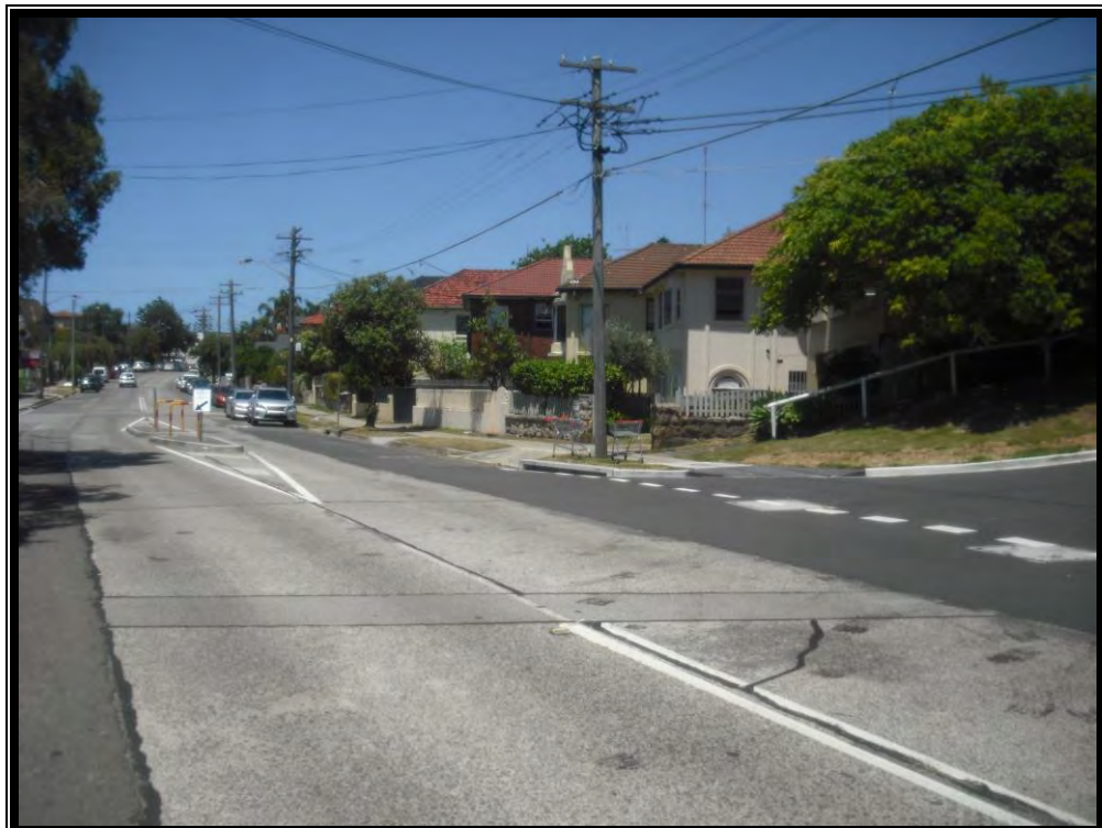
Photo 2: the frontage of the subject site to Old South Head Road
