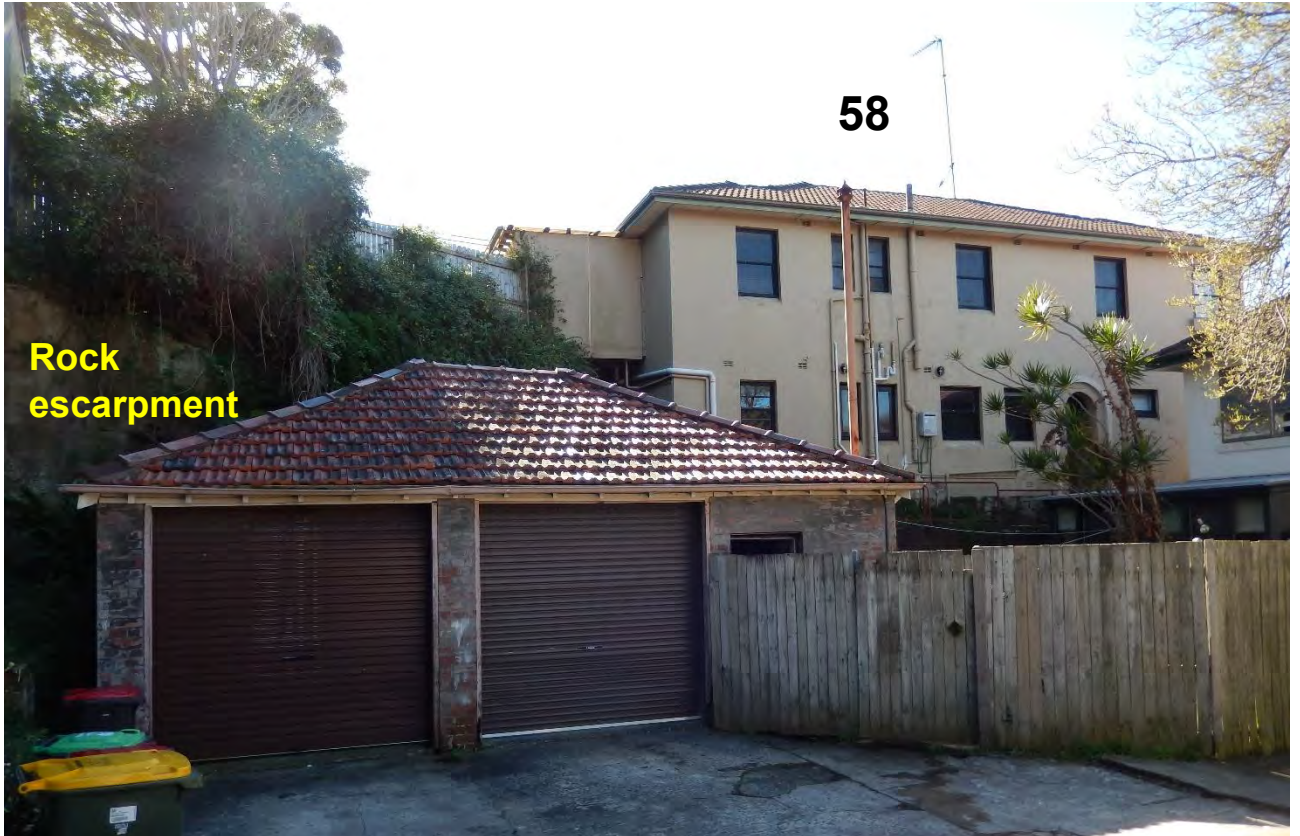
Figure 13: Existing development at 58 Old South Head Road seen from the rear yard of 56 Old South Head Road, showing rock escarpment to the left
