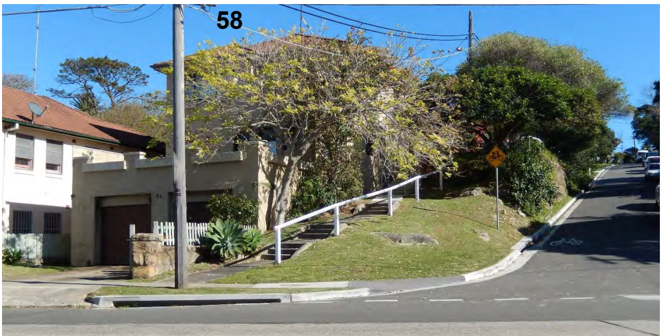
Figure 12: Existing development at 58 Old South Head Road showing Clarendon Street, public stairs and steep topography of site and surrounds
