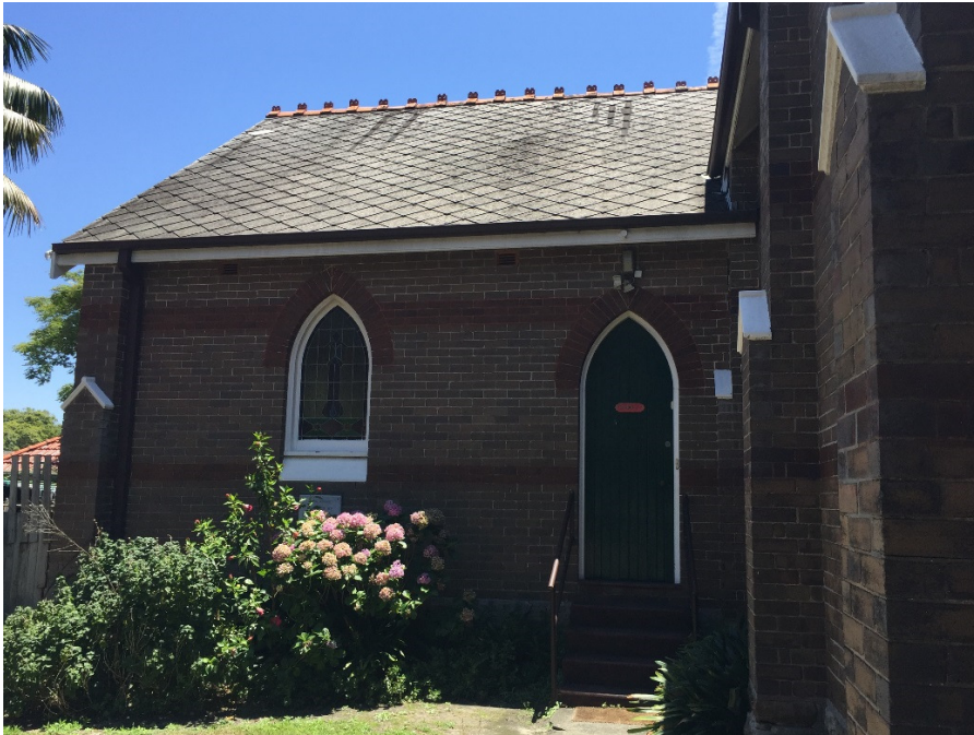
Figure 4.13 – View of Classroom alterations 1924 (Source: RA Moore February 2018)
