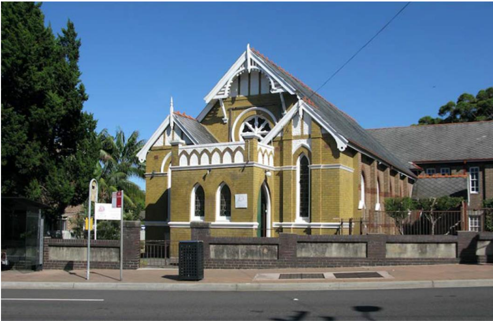
Figure 1: Rose Bay Methodist Church (1904) and the Wesley Hall (1929), (Source: RA Moore February 2018).
