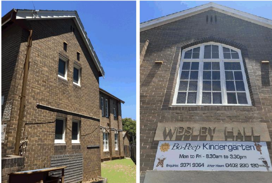
Figure 4.18 Rear Elevation and Principal façade Wesley Hall (Source: RA Moore January 2018)
