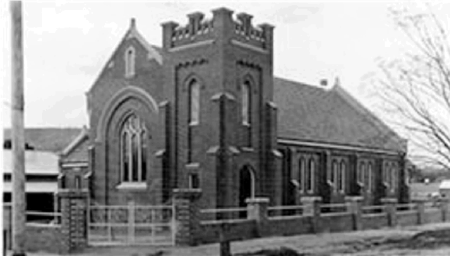
Figure 5.1 Bowral Methodist Church (Now Uniting), 1881. Bendooley Street, Bowral. (Source: http://bkuc.com.au/history/ 10 February 2018).
