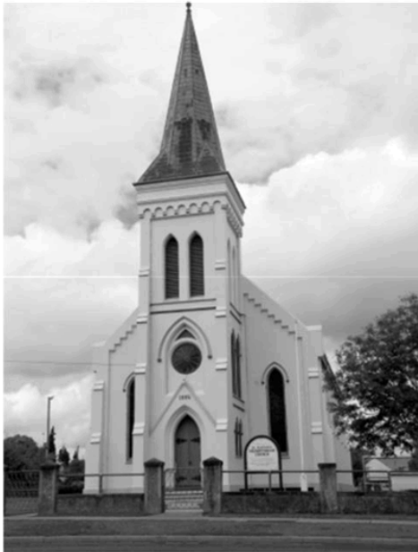
Figure 5.2 St Andrews Presbyterian Church, Grafton NSW, 1885. (Source: http://mapio.net/pic/p-6790838/ 10 February 2018)
