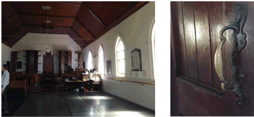
Figure 4.2 Church interior, door furniture (Source: RAM February 2018)
