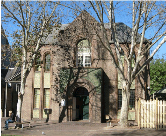
Figure 5.3. George Smith Memorial Hall, Paddington Methodist [Uniting Church] Oxford Street, 1919 (Source: Michael Bogle).
