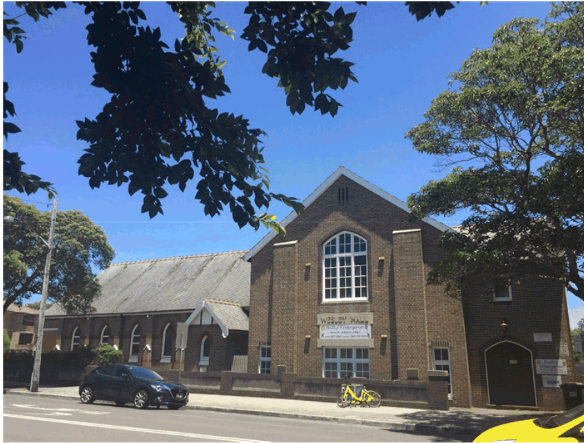
Figure 4.4 Wesley Hall and North elevation of Church from Dover Road (Source: RA Moore, February 2018)
