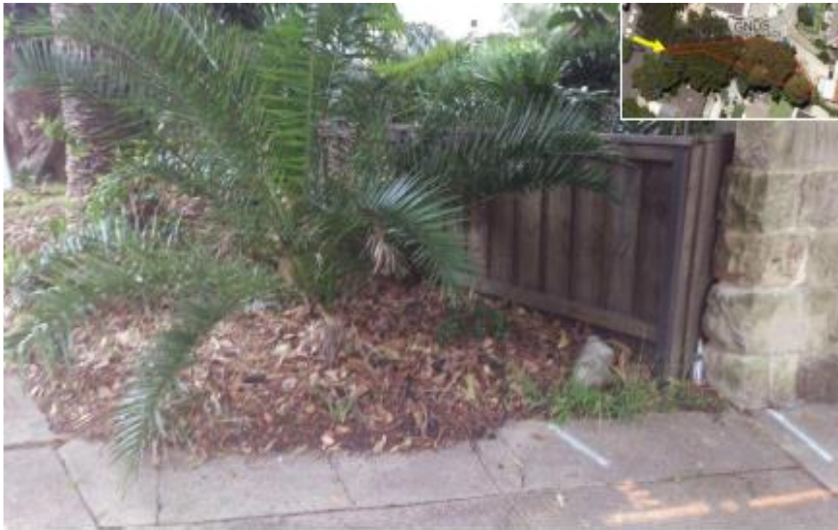
Figure 6: Photograph of the 2.7m wide Council and public access to the site from Wentworth Street. This is the only legal access to the site.
