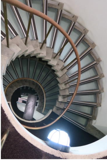
Figure 26.0, Showing later light fitting and original metal bracket for securing Kitching Sculpture.
