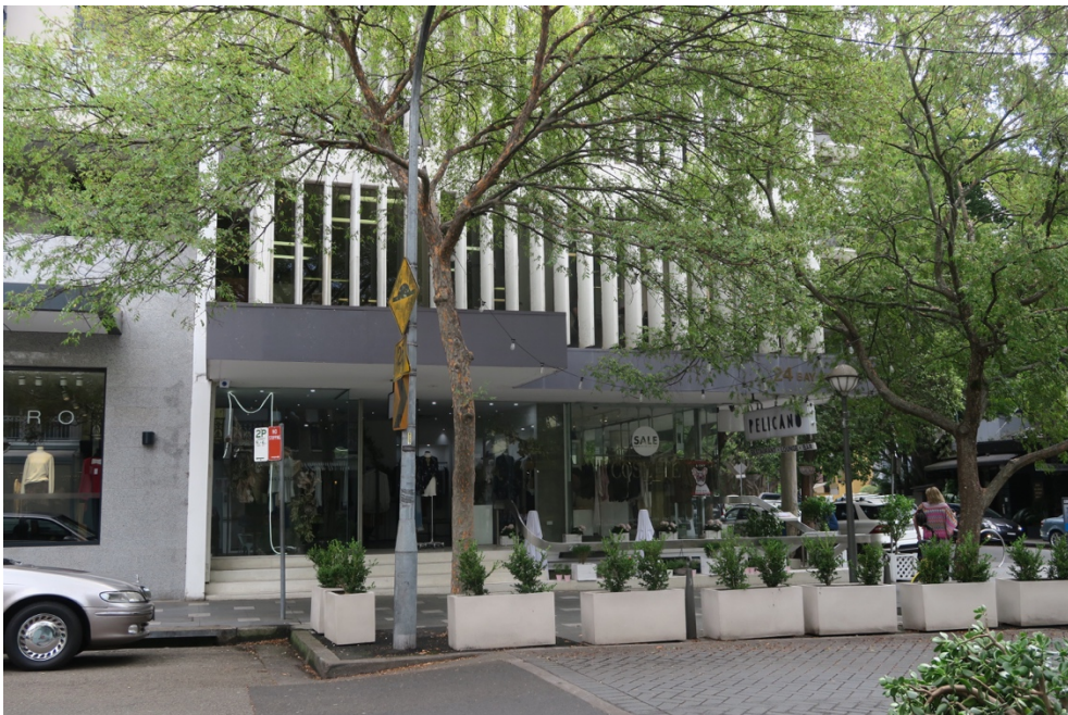
Figure 13.0, Bay Street elevation showing generous articulation of the corner provided by the shop set-backs, the podium and the spacious corner area devoted to stairs to basement restaurant, giving a sense of openness to the corner. There is no gratuitous or superfluous detailing – all is refined and purposeful.
