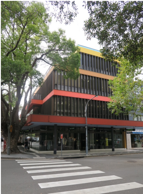
Figure 66.0, Corner Bay St and Knox St
