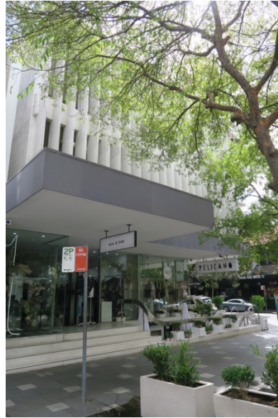
Figure 15.0, East façade with vertical louvres
