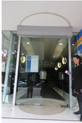
Figure 19.0, Terrazzo paving demarcating original location of automatic door.
