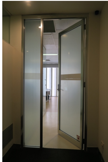
Figure 39.0, Entrance to upper level office, showing original aluminium frames and full height door with frosted glass.
