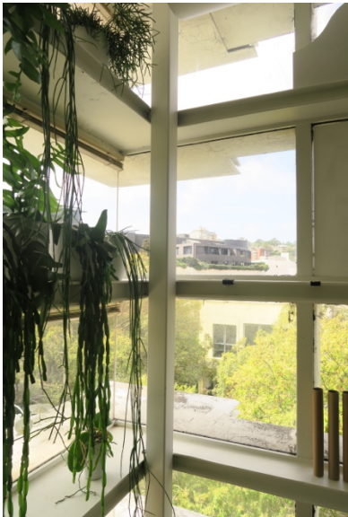
Figure 38.0, Corner window detail. There are no opening windows in the building – to maintain the clean lines of the exterior.
