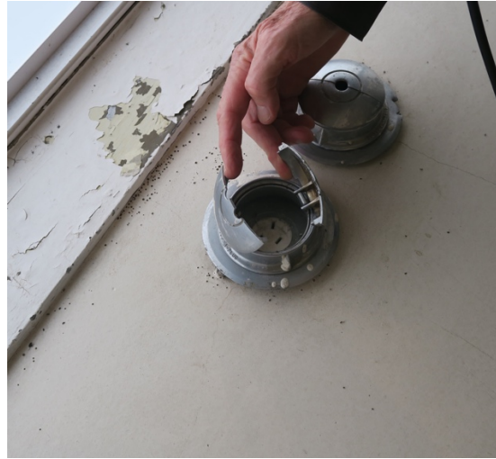
Figure 37.0, Original concealed floor mounted power-points in upper level office.
