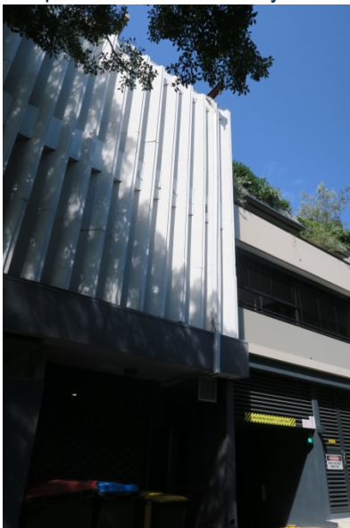
Figure 16.0, West façade angled louvres.
