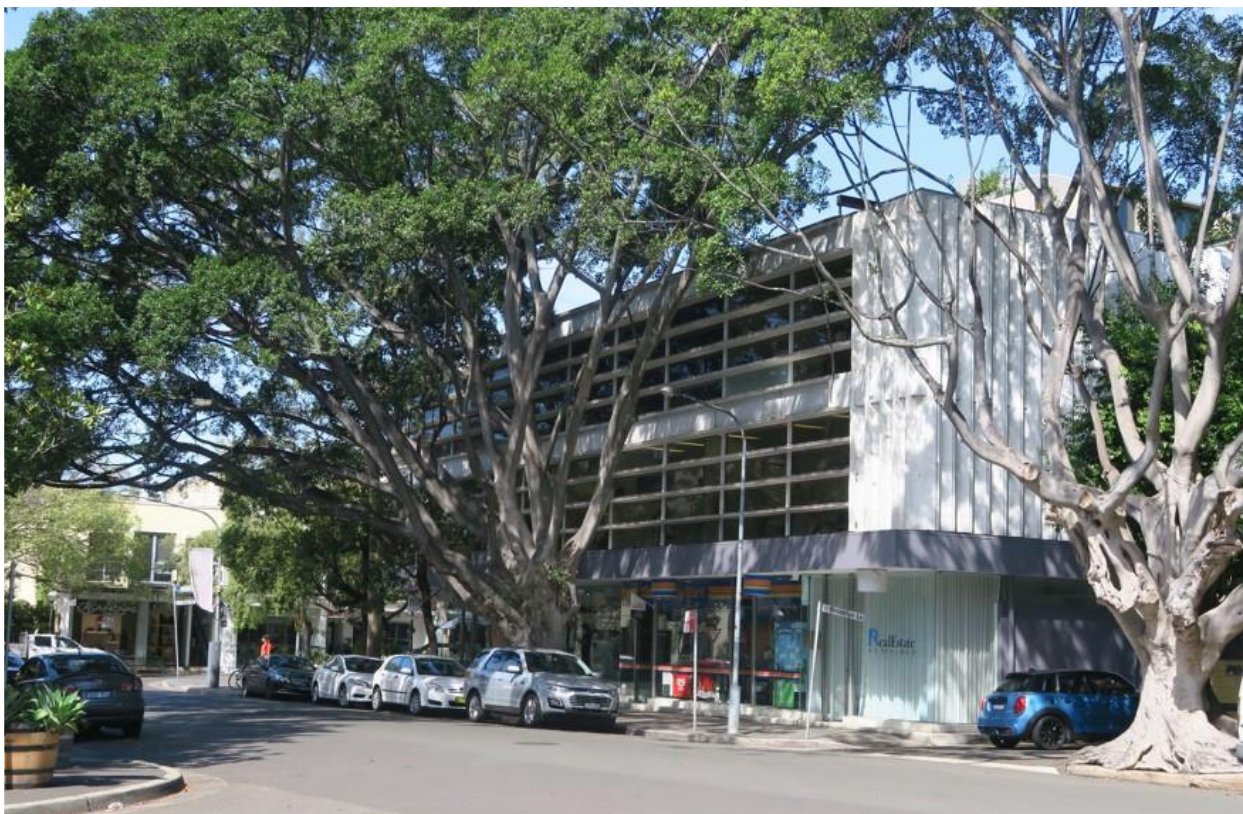
Figure 1: Gaden House viewed from South Avenue, looking towards north and west elevation and Brooklyn Lane (Source: Anne Warr Heritage Consulting 20 June 2018)
