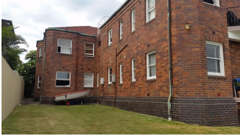
Figure 9 – Existing Development – 636 New South Head Road Source: JBA
