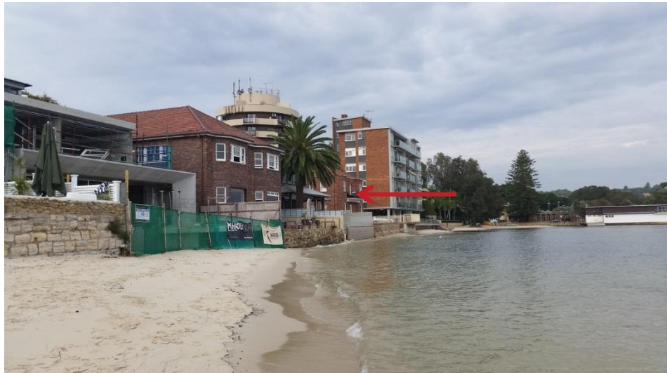
Figure 10 – Existing Development – 636 New South Head Road Source: JBA
