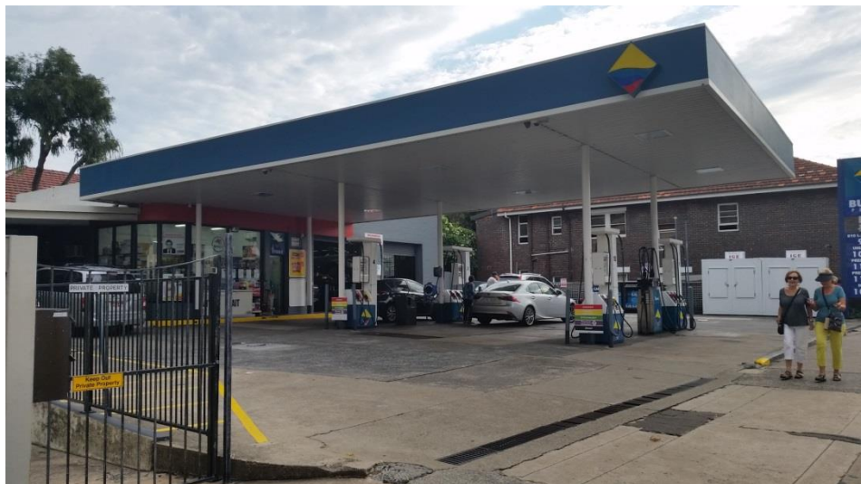
Figure 11 – Existing Development – 638 New South Head Road Source: JBA
