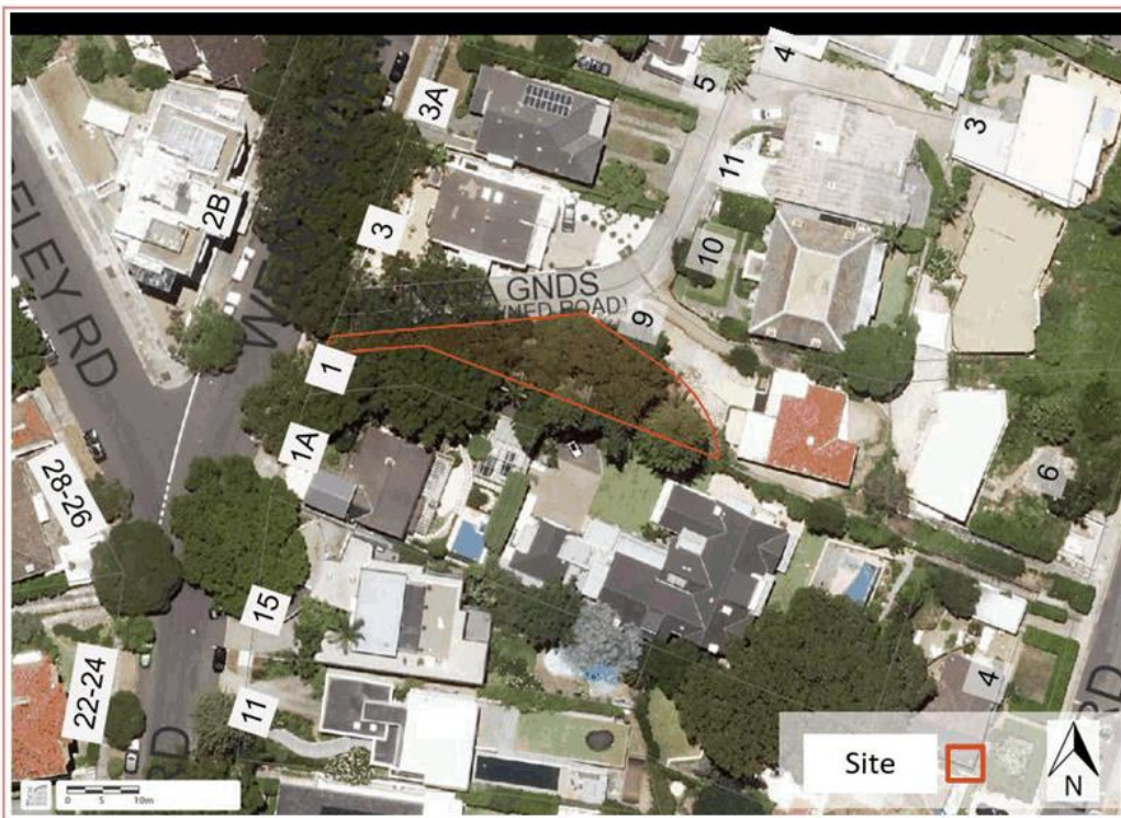
Figure 3 Aerial photograph showing the subject site outlined in red
