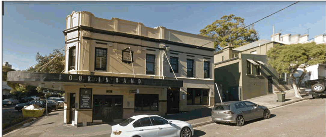
(Source: Google Street view – July 2017)
