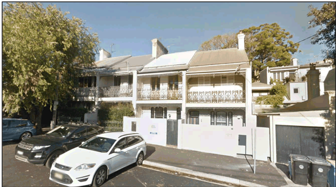
(Source: Google Street view – July 2017)
