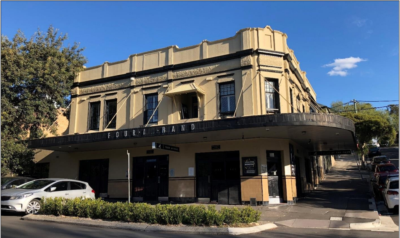
Figure 1: The Four In Hand Hotel as viewed from Sutherland Street, looking towards the north eastern and north western elevations
