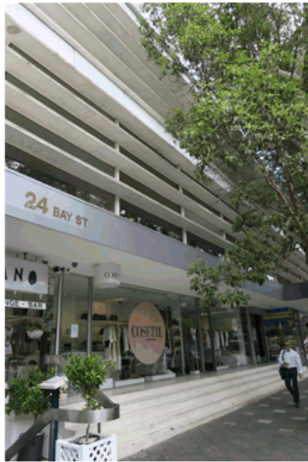
Figure 14.0, North façade with horizontal louvres to the office space which seem to float above the long run of horizontal podium. The long flight of stairs reflects the horizontal louvres above, combining to create a composition in horizontality.
