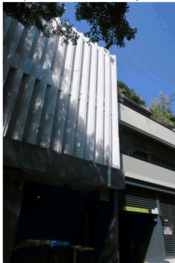
Figure 16.0, West façade angled louvres.
