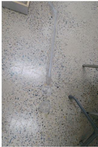
Figure 40.0, Level one terrazzo floor showing markings from former partition system
