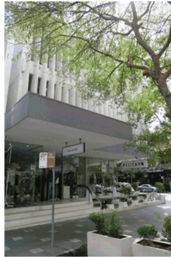
Figure 15.0, East façade with vertical louvres
