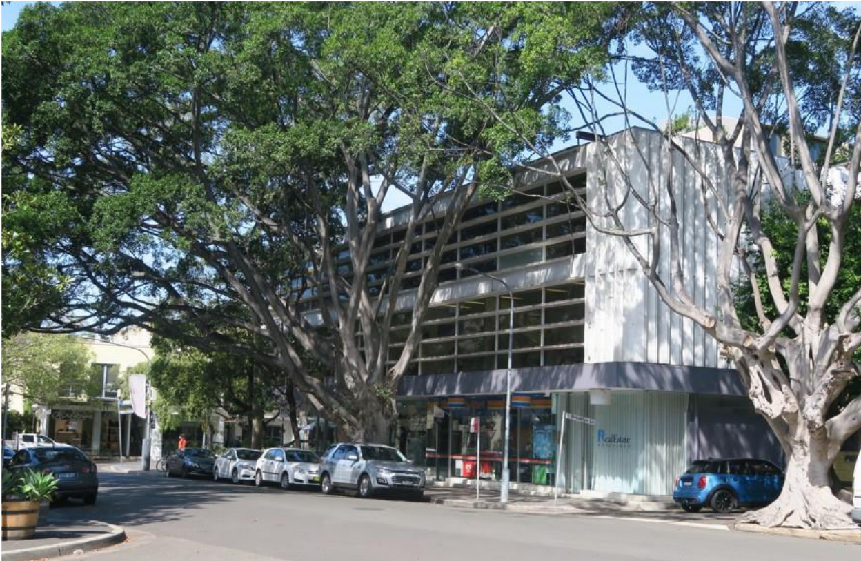
Figure 1: Gaden House viewed from South Avenue, looking towards north and west elevation and Brooklyn Lane (Source: Anne Warr Heritage Consulting 20 June 2018)
