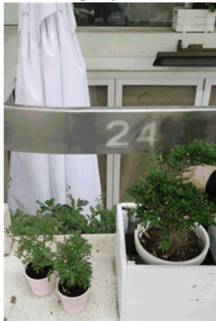
Figure 20.0, Street number inset into handrail
