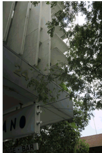
Figure 17.0, Junction of east façade and northern louvres, creating an egg-crate effect.
