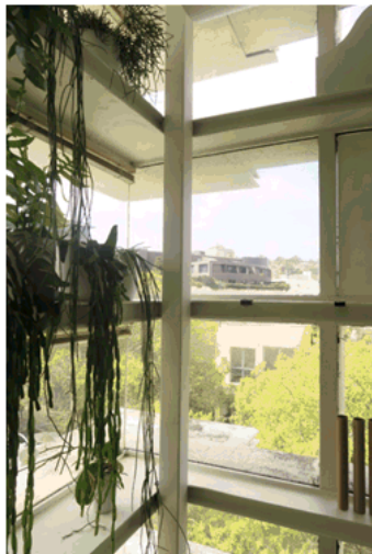
Figure 38.0, Corner window detail. There are no opening windows in the building – to maintain the clean lines of the exterior.
