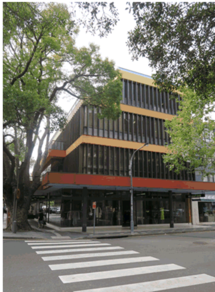
Figure 66.0, Corner Bay St and Knox St
