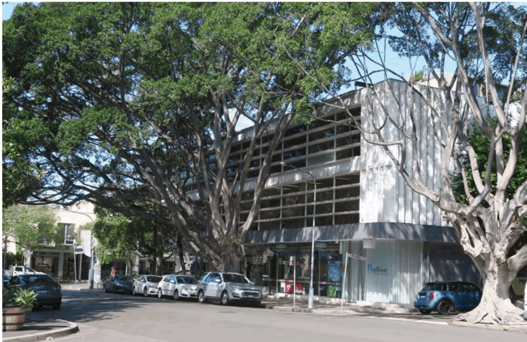
Figure 1: Gaden House viewed from South Avenue, looking towards north and west elevation and Brooklyn Lane (Source: Anne Warr Heritage Consulting 20 June 2018)
