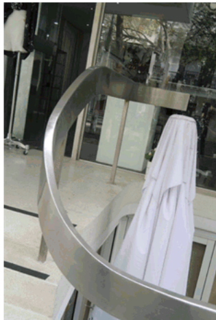
Figure 18.0, Handrail leading to Shops 2 and 3 facing Bay Street.
