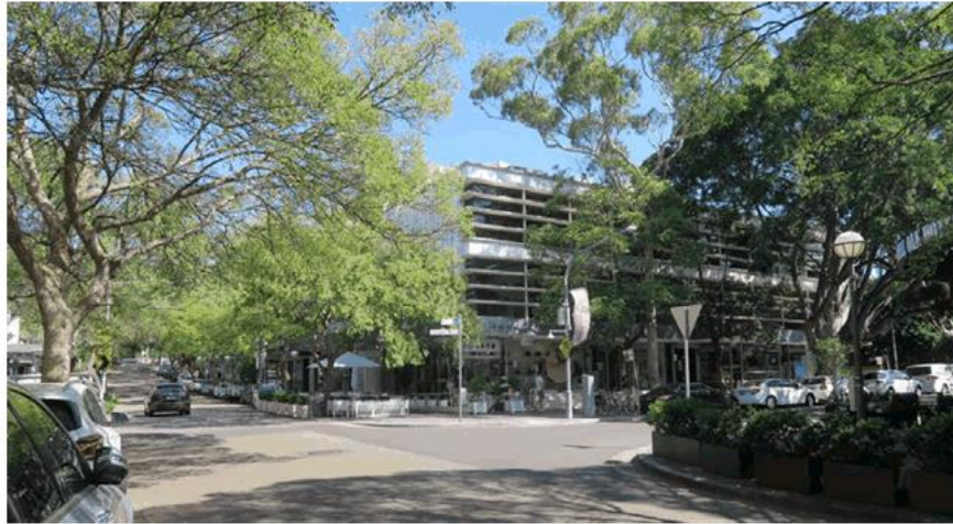
Figure 9.0 The subject building viewed from the corner of Cooper and Bay Streets, Double Bay. Note the horizontal louvres facing Cooper Street and the vertical louvres facing Bay Street.
