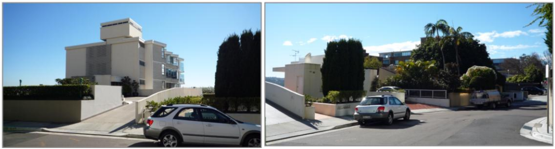
Figure 14: Photos of Nos. 73-75 Yarranabbe Road (left) and Nos. 77-81 Yarranabbe Road (right). These apartment buildings feature vehicular access points off Yarranabbe Road with car lifts within the building forms to access the car parking areas on the levels below. The building forms are orientated to the Harbour views to the north (Source: CPSD)
