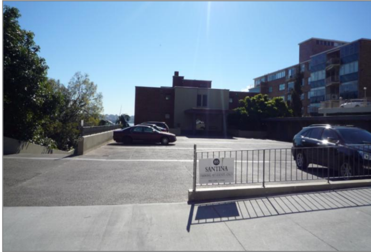
Figure 12: View of the adjoining residential building to the east, 'Santina,' No. 85 Yarranabbe Road showing the vehicular access and parking area which dominates the street setback and adjoins the boundary of the subject site (left). The combination of the car park on the adjoining property and the car ramp on the subject property degrades the quality of the public domain in this part of Yarranabbe Road (Source: CPSD)
