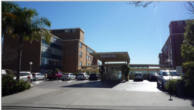
Figure 13: View of the apartment building to the east, Nos. 87-97 Yarranabbe Road, showing the vehicular access and parking area which dominates the street setback of the apartment building and the pedestrian experience on this part of Yarranabbe Road (Source: CPSD)
