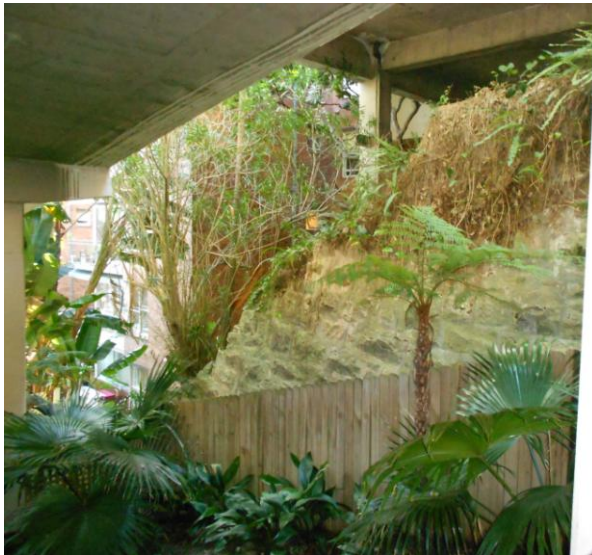
Figure 17: Photo taken from beneath the raised driveway ramp of the subject site looking towards 'Santina.' This area consists of substantial structural features including the raised driveway and parking structures of the subject site and Santina, as well as the substantial 'rockery' retaining structure (right) (Source: Tzannes Associates)
