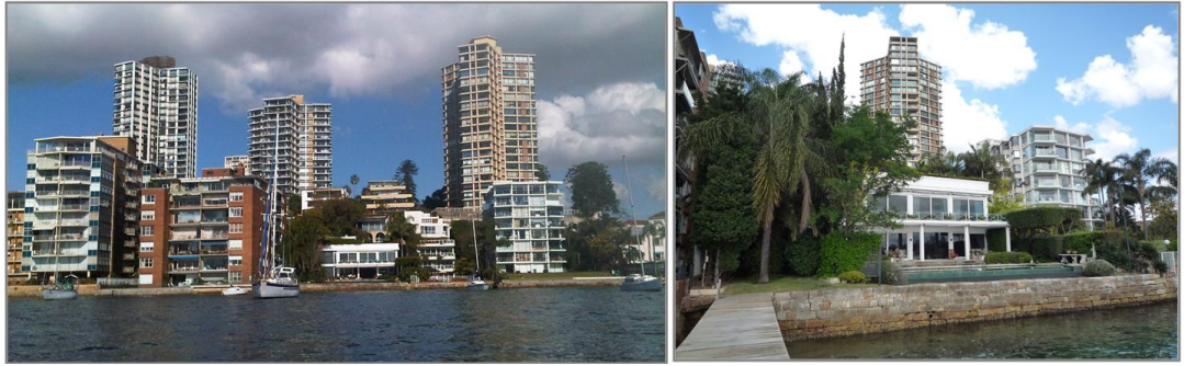
Figure 4: Photos of the site as viewed from the Harbour. The dwelling house at No. 83A Yarranabbe Road comprises a two level dwelling comprising 4 bedrooms and a swimming pool. The rooftop parking is accessed by a raised driveway along the eastern boundary of the site. The portion of the site which accommodates the dwelling at No. 83A is relatively flat.
