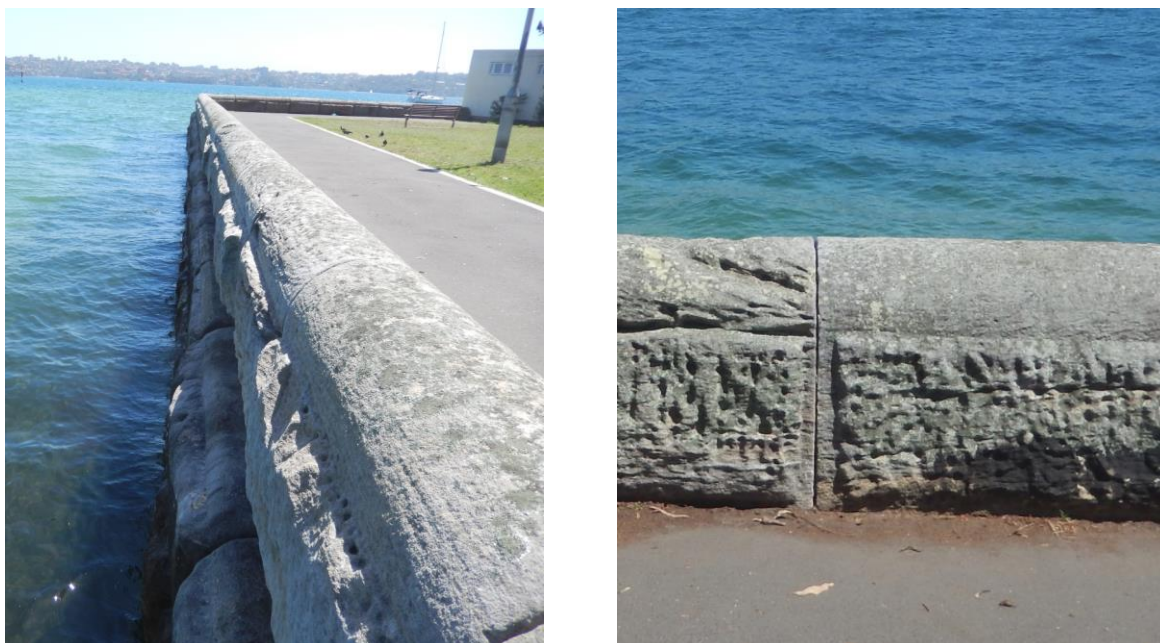
Figure 2. Photographs of the seawall
