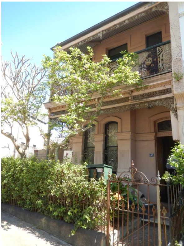
Figure 2. Front façade of 48 Duxford Street, Paddington
