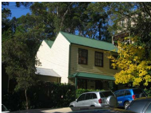
Figure 3 Double transverse gable roof form, Harris St, Paddington
