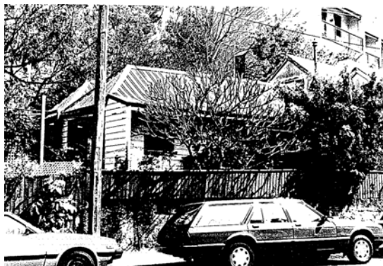
Figure 4 Double transverse hipped roof form
