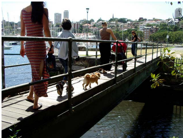
Figure 1 displays the narrowness of existing bridge across stormwater canal.
