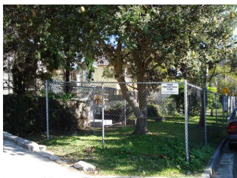
Figure 1. A typical example of chainmesh fencing and signage to be installed as fencing for tree protection zones.
