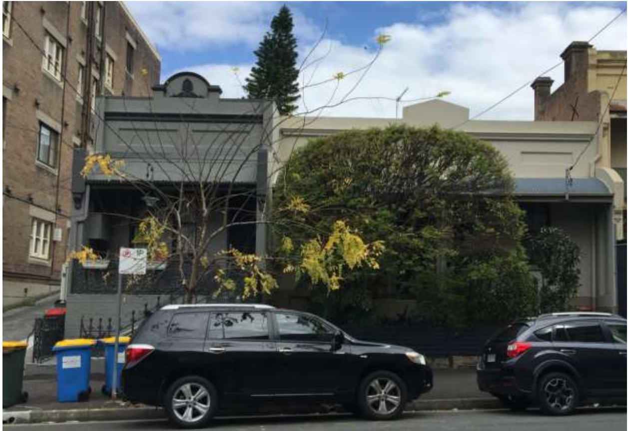
Figure 3: Existing single storey terraces at 190-194 Boundary Street (source SJB)
