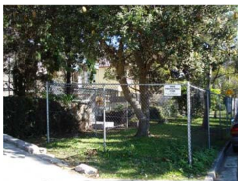
Figure 1. A typical example of chainmesh fencing and signage to be installed as fencing for tree protection zones.
