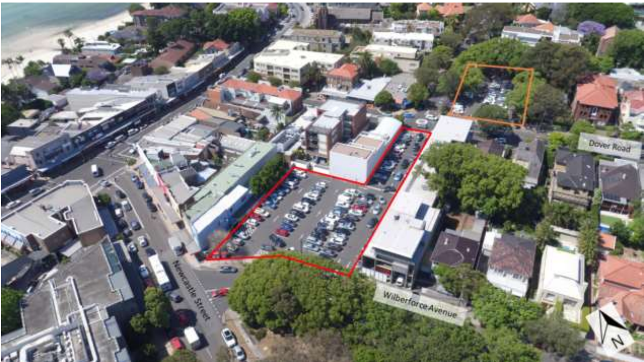
Figure 4: Oblique aerial of the Rose Bay Centre
