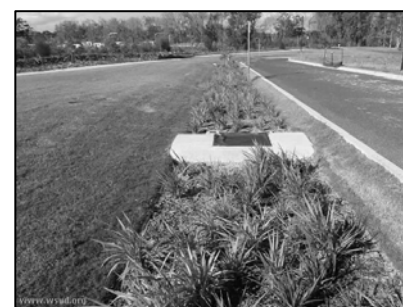
Photograph 1 Typical roadside bioretention system with grass buffer strip
