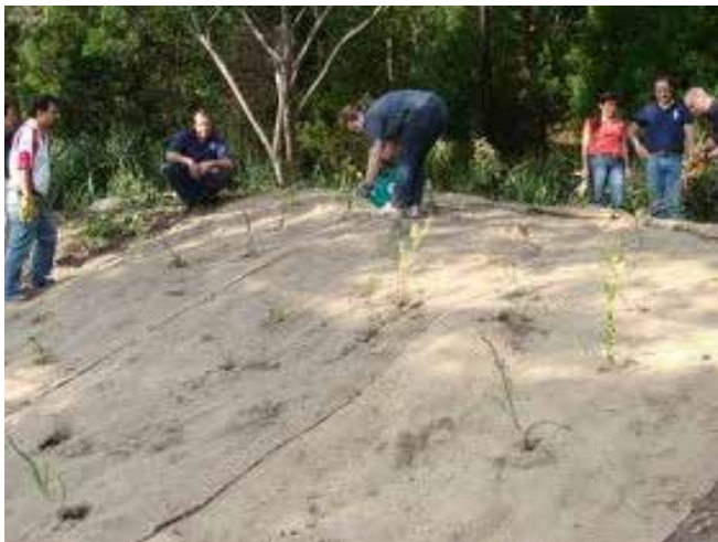
Figure 28. Bushcare volunteers and staff completing planting out on a stabilised slope in Trumper Park
