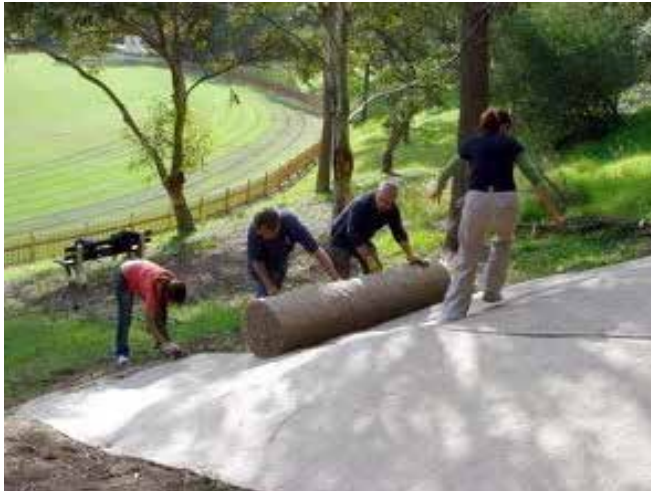
Figure 27. Bushcare volunteers assisting staff to stabilise steep slopes in Trumper Park prior to planting
