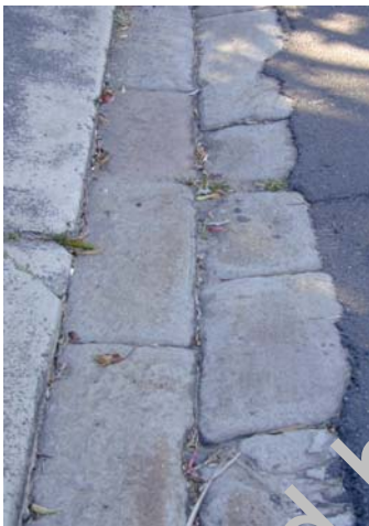
Figure 5.7 Sandstone guttering.
