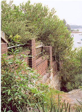
Figure L.7 Composite wall containing sandstone and face brick on Salisbury Street.
