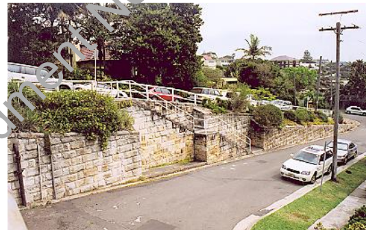
FIGURE 91 Significant sandstone retaining wall
