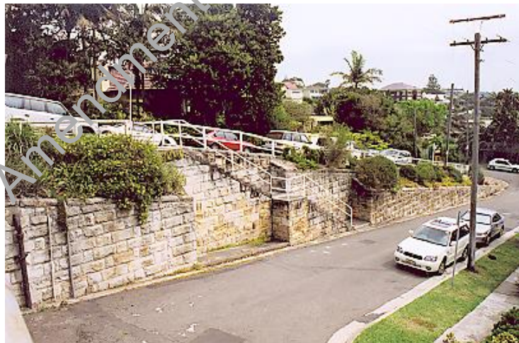
Sandstone retaining wall along Salisbury Street
