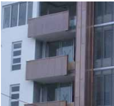
FIGURE 3 Part projecting balcony
