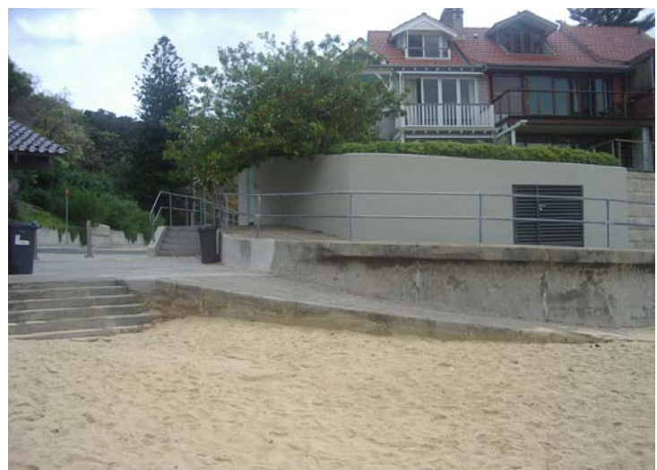
Existing access ramp at Camp Cove Beach
