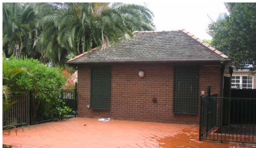
Photograph 4: The existing garage on the subject site.
