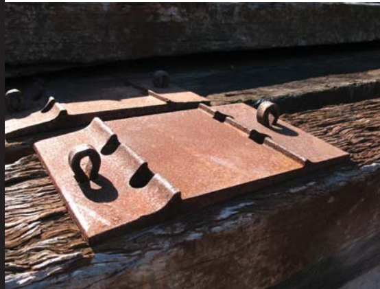
Tram infrastructure, 2007 Source: Sydney Tramway Museum, TBLD
