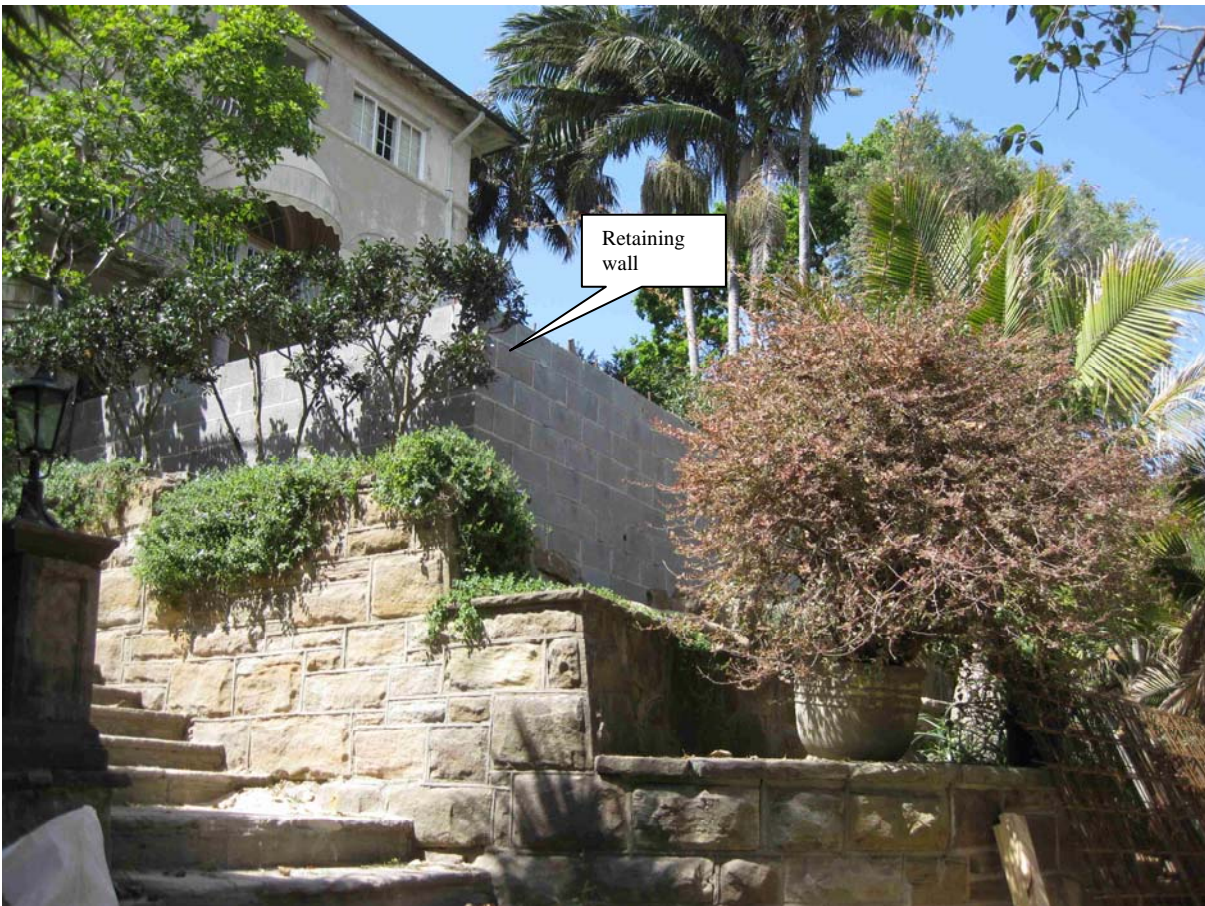
Photo 2 -view of north west section of retaining wall
