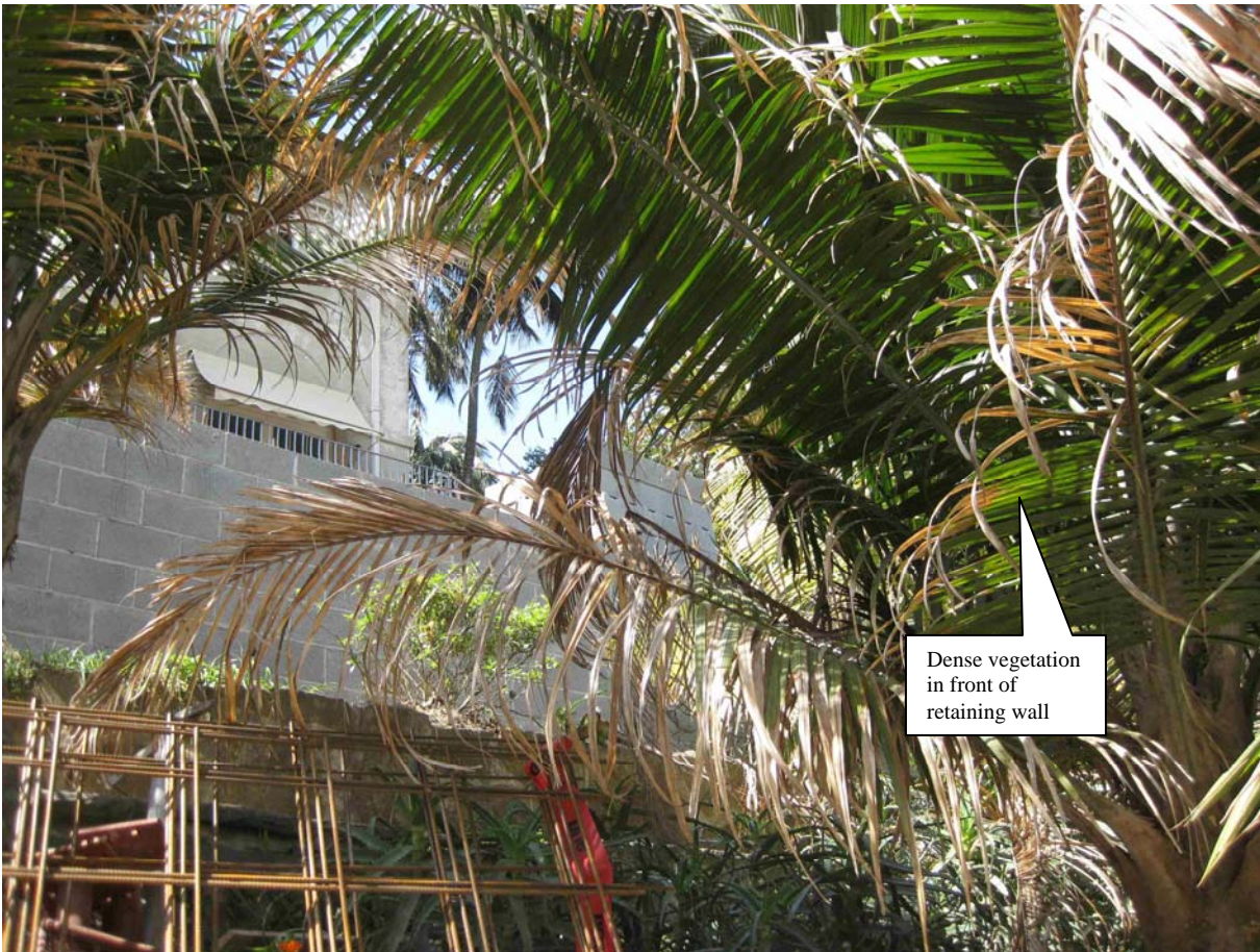
Photo 3 -view of western section of retaining wall
