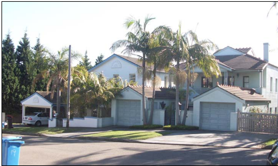
No. 18 and No. 20 Chamberlain Avenue
