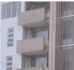
Fig 5.6 Part projecting balcony
