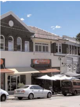
Fig 5.7 98B Bellevue Road at Streatfield Centre
