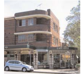
Fig 5.4 Strong corner building - Plumer and O'Sullivan Roads
