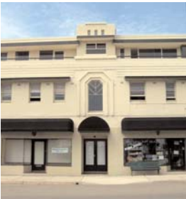
Upper level entry, South Head Roundabout
