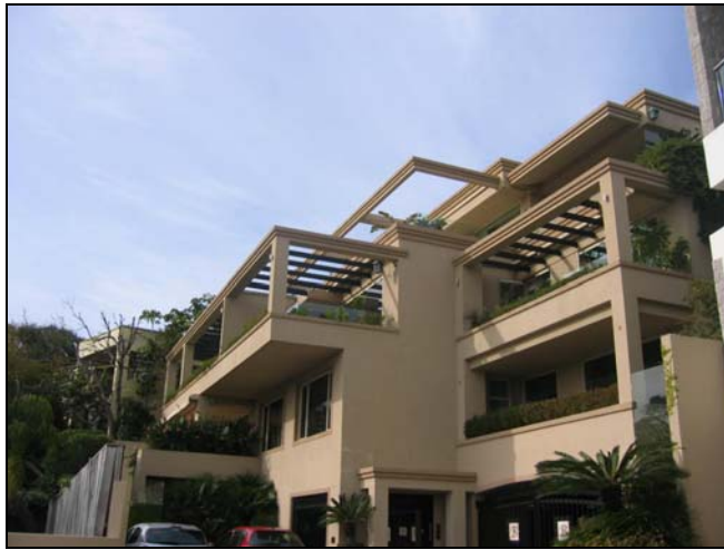
i) The subject second floor balconies at units 2 & 3/18 Ian Street – viewed from the front drive.
