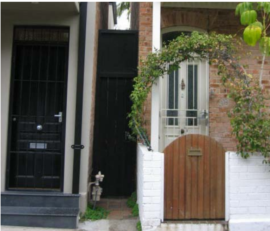
View 9: View of gate between No. 33-35 located within the street front zone and forming part of the principle elevation of both terraces.
