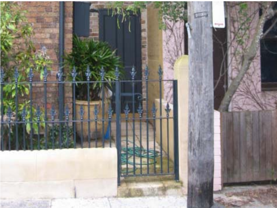
View 7: View of bricked up former rear lane access to no. 31 Dudley Street Paddington, located within the street front zone and forming part of the principle elevation.
