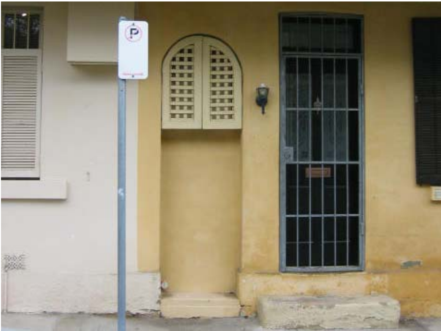
View 10: View of bricked rear lane access to no. 39 Dudley Street Paddington, located within the street front zone and forming part of the principle elevation.
