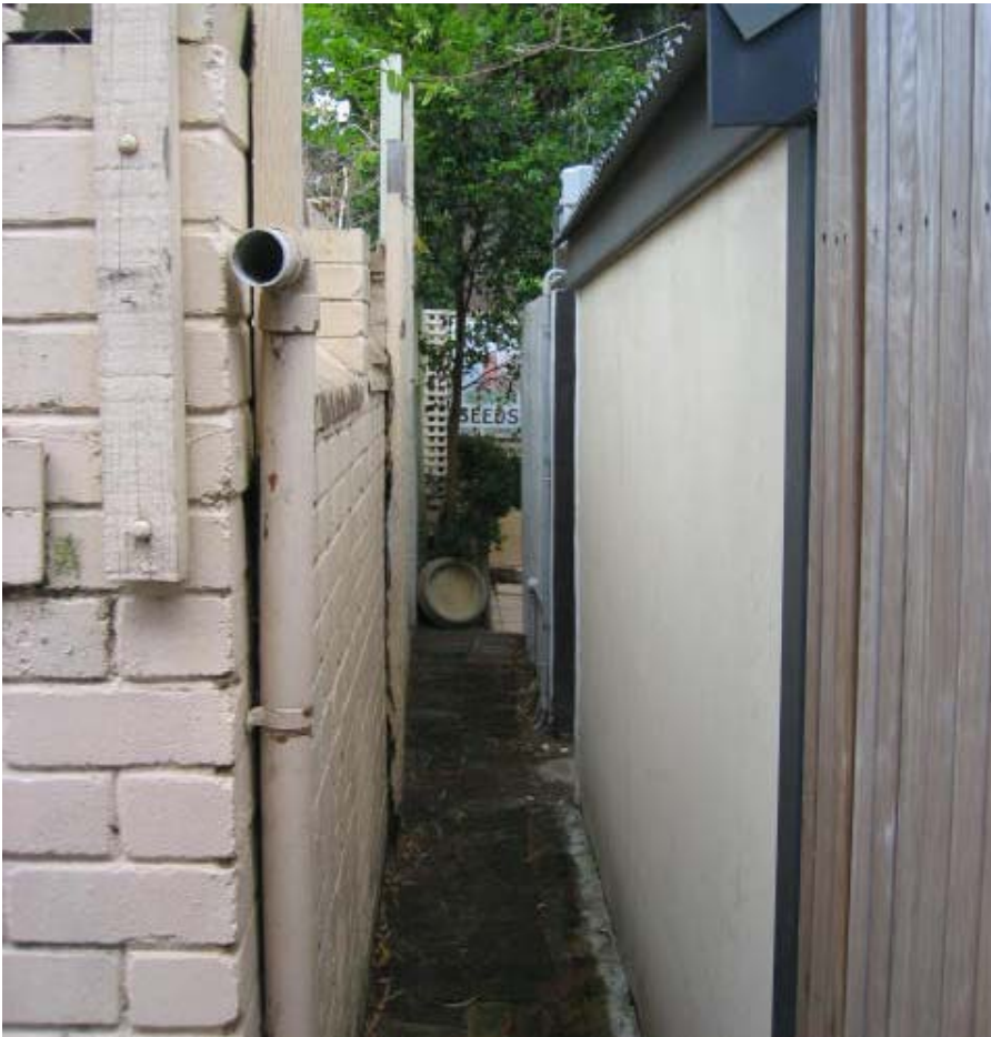
View 2: View of rear of subject site, showing that the former night soil lane behind nos. 7-15 Dudley Street and nos. 93 – 101 Underwood Street has now been substantially enclosed. The subdivision pattern suggests that the original passage would have extended east to 15 Dudley Street and 101 Underwood Street.
